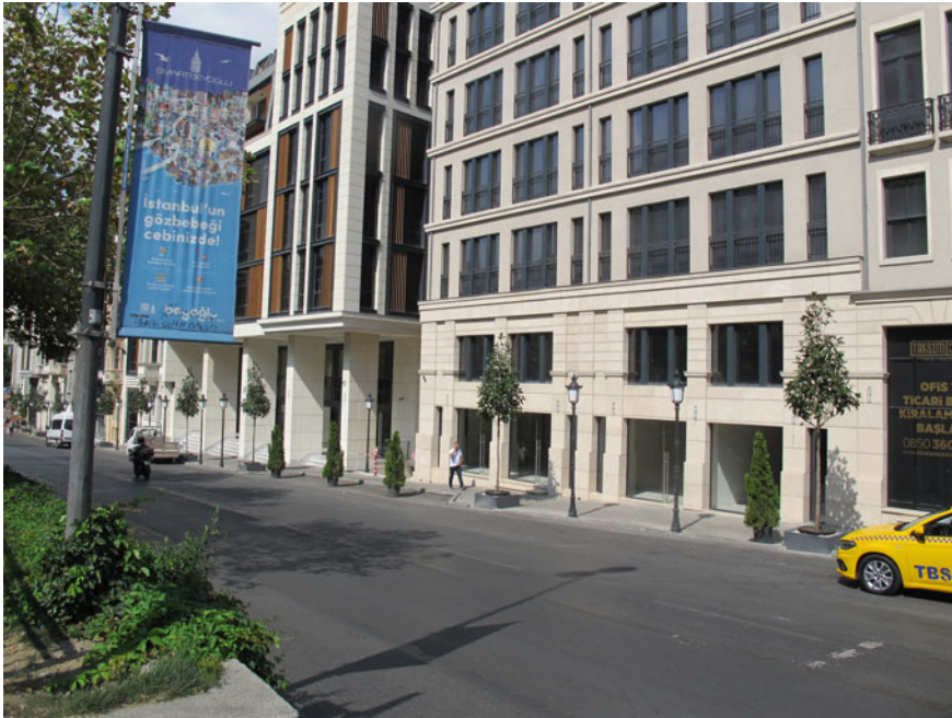
Fig. 12.12 Tarlabasi Renewal Project, Beyoğlu ( Source Image by authors )
