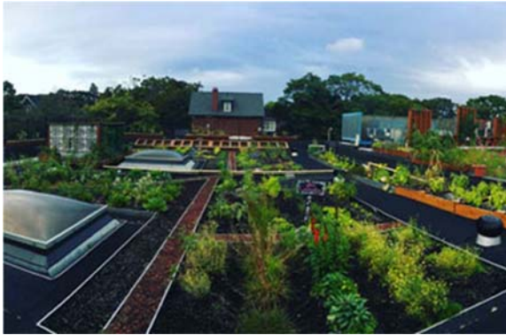
Figure 4.9 Example of a green roof (source: greenroofs.org).
