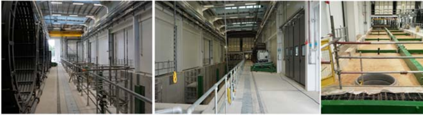
Figure 9.4 Upstream and downstream view of the full experimental facility constructed at ICAIR, plus a detailed view of a full-scale manhole. ©The University of Sheffield and ©SimonTait.
