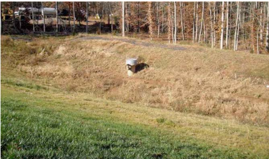
Figure 4.1 An example of an infiltration basin which can fill to the invert of the outlet structure (source: www.rivanna-stormwater.com ).
