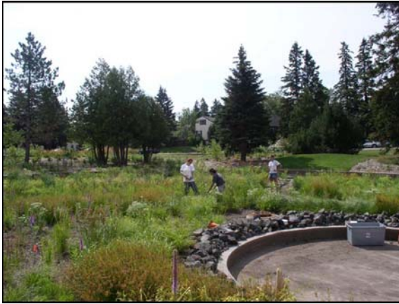
Figure 4.6 Bioretention facility draining parking lot (photo by authors).
