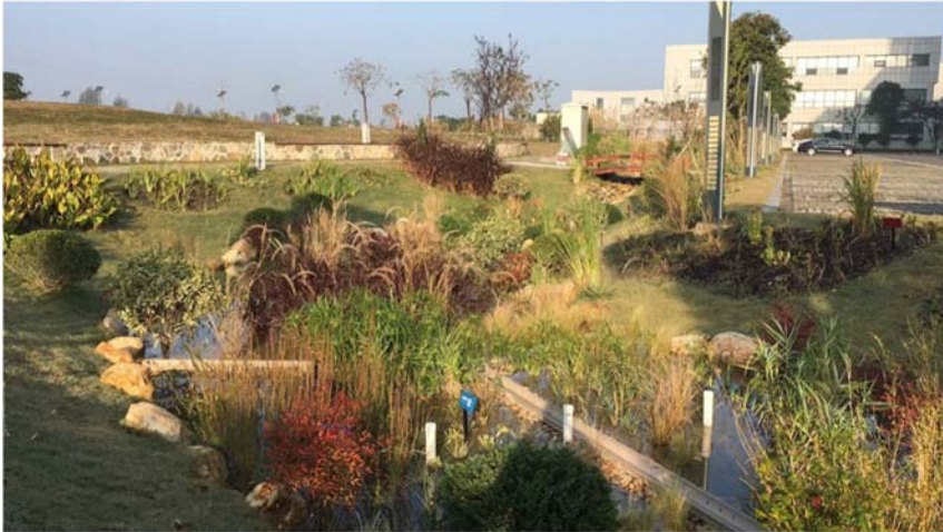
Figure 5.4 Picture of the biofilter system taken in September 2018 immediately after a rainfall event.
