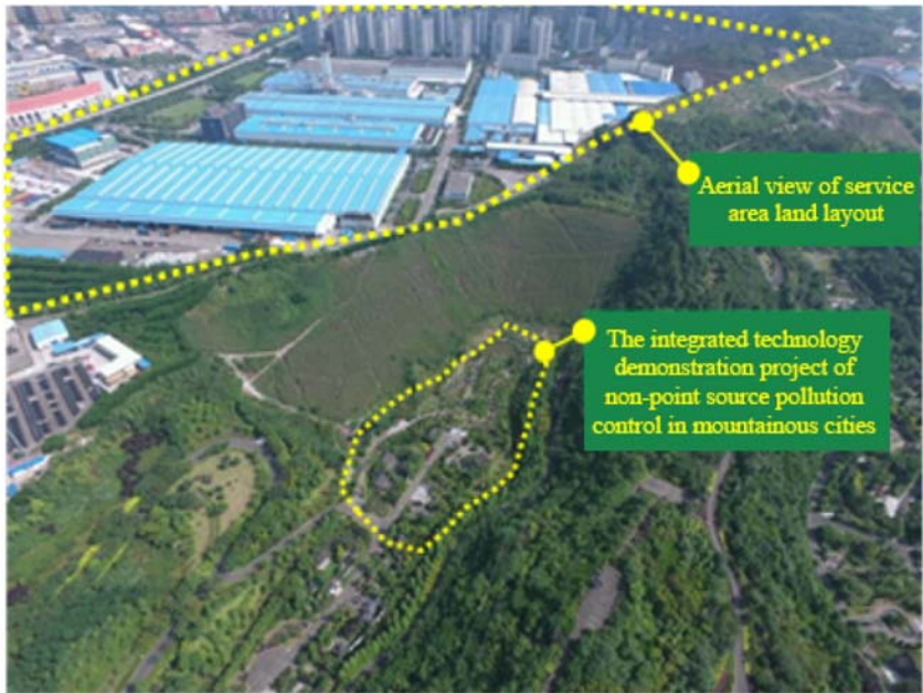
Figure 13.5 Aerial view of the integrated technology demonstrative project (photo by authors).
