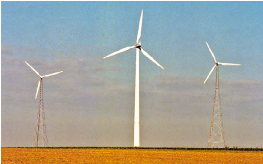
Figure 2.25: Subjective visibility comparison between conventional tubular steel tower and lattice towers. Photo: Sinning and taken from Hau [93, p. 520]
