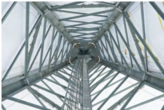
Figure 2.21: View into the pentagonal space frame lattice tower of GE [78]
