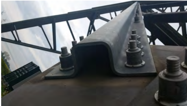
Figure 2.24: Lockbolts of the Butzkies tower and diagonal member with hat cross section. Photo: A. Struve 2018
