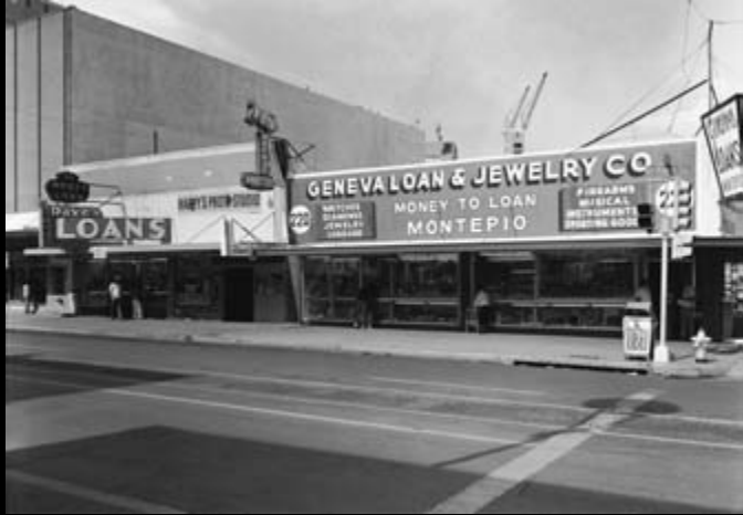
South El Paso St., 216–222, El Paso, Texas, 1980. Photograph by David Kaminsky, Library of Congress, Prints and Photographs Division, HABS TEX, 71-ELPA, 4-14.
