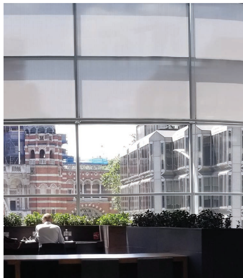
Figure 18.1 Window shades half closed all day without changes to control the amount of daylight
