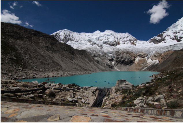
[Fig. 2] Panoramic view of Lake Palcacocha from one of its dams. On the left side: part of the early-warning system installed in 2019. At the center: rubber pipes used to drain the water from the lake (Source: Usón 2020)
