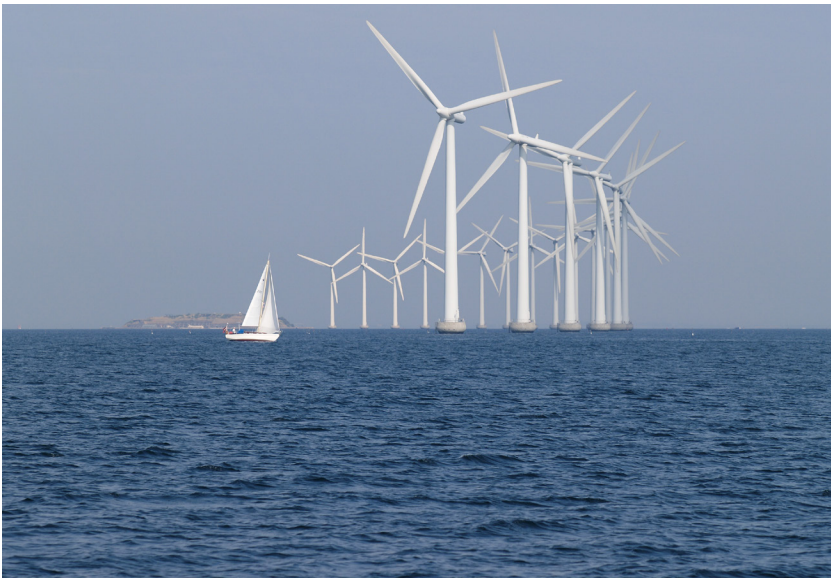
Figure 1.2: Middelgrunden Offshore Wind Park, Denmark.
