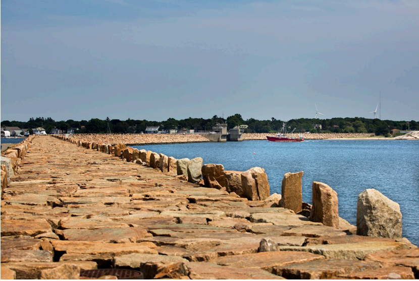
Figure 6.3: New Bedford, MA, USA, hurricane protection barrier, completed in 1966. The barrier is located in New Bedford and Fairhaven Harbor, approximately 50 miles south of Boston. The project protects about 1,400 acres (567 hectares) in the towns of New Bedford, Fairhaven, and Acushnet.
