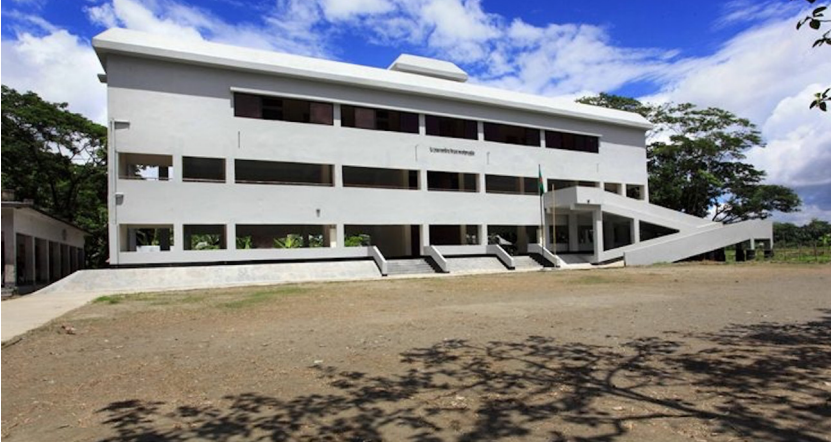
Figure 6.6: Uttar Seral Government Primary School, Agulchara, Barishal, Bangladesh. The building is also a cyclone shelter.
