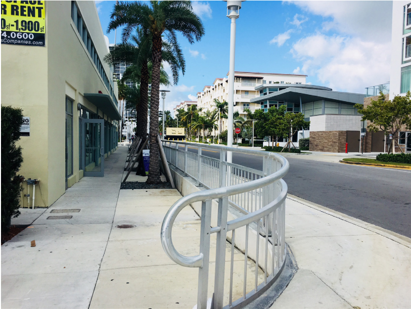
Figure 6.4: A raised road in the city of Miami Beach, Florida. The elevation acts as a defense against flooding.
