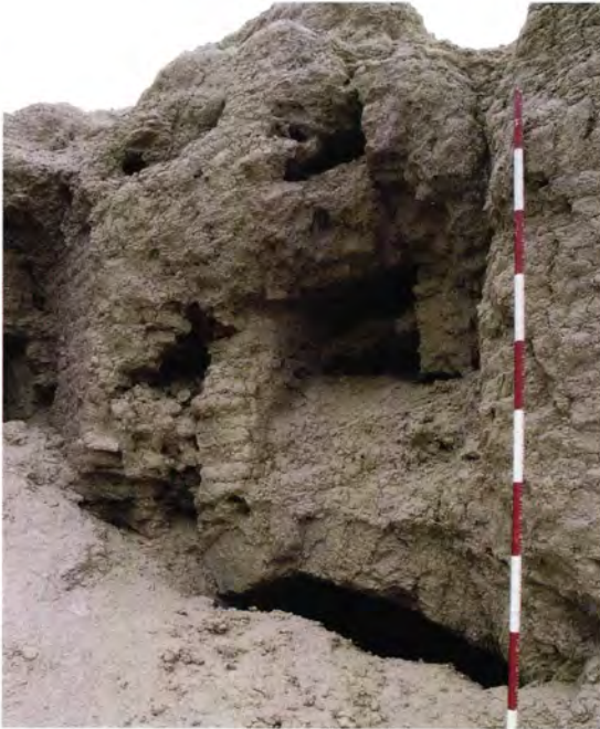
Figure 234 Kyz Kala [13] near Kelte Minar: detail of the collapsed north corner with the top of the vault of the stairway, 8. The vault was reinforced with ribs or armatures.
