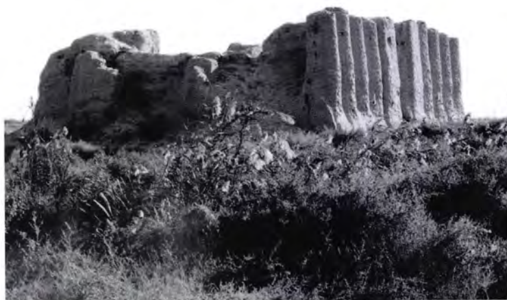
Figure 232 The south-west and collapsed north-west façades of Kyz Kala [13] near Kelte Minar. Note the flattened pilasters in the centre of the south-west façade, and the corrugations starting from near the ground.
