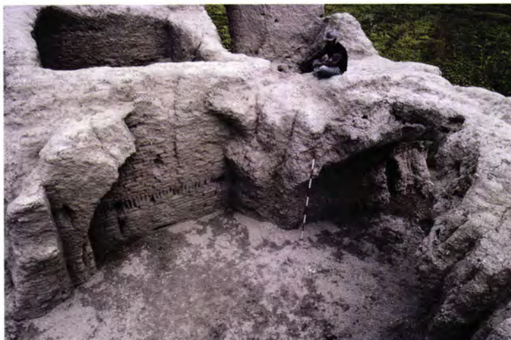
Figure 251 Yakkiper Köshk [17]: a view into the cruciform Room 2 from the upper storey. Note the vaulting of the internal arches and the band of brick laid vertically.
