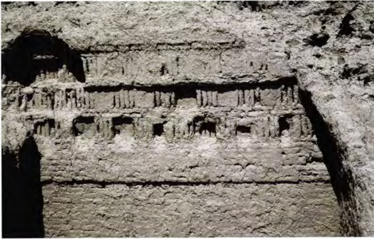
Figure 263 The palace in Shahryar Ark [20]: 'chequerboard' brickwork in the back wall of Room 17, framed by the walls of the vault and set above a deep string course.
