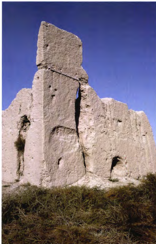
Figure 248 The east façade of Yakkiper Köshk [17]. The walls are plain, relieved only by a string course of fired bricks between the second and third storeys: there is a low door (see Figure 249) in the centre.
