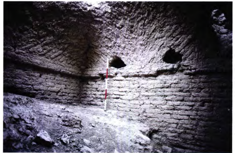
Figure 254 Yakkiper Köshk [17]: Room 8, roofed with a squinch or balkhi vault on a string course, with triangular slots.
