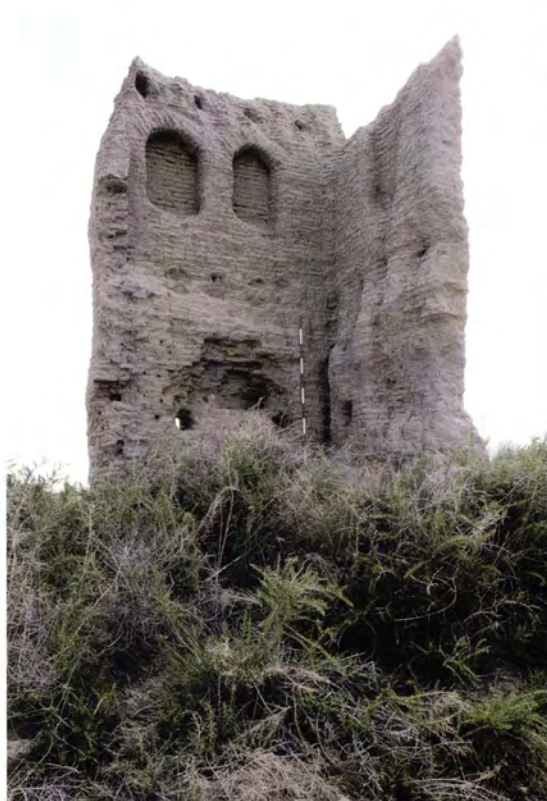
Figure 311 The interior of Electricity Station Ding 3 [32c], a two-storey ding with niches on both floors.
