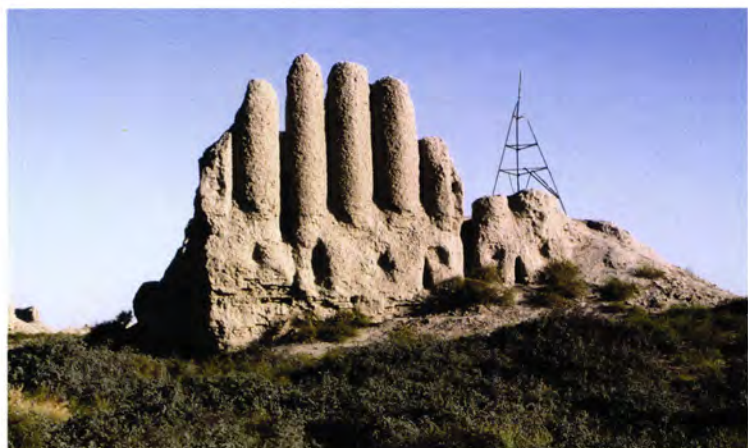
Figure 219 View of Byash Barmak Köshk [8] from the south west, the only köshk surviving within a city.
