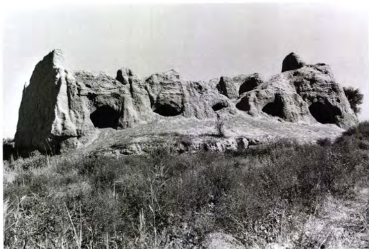
Figure 203 Byash Ishyk Köshk [5]: the vaulted rooms behind the collapsed north-west wall.
