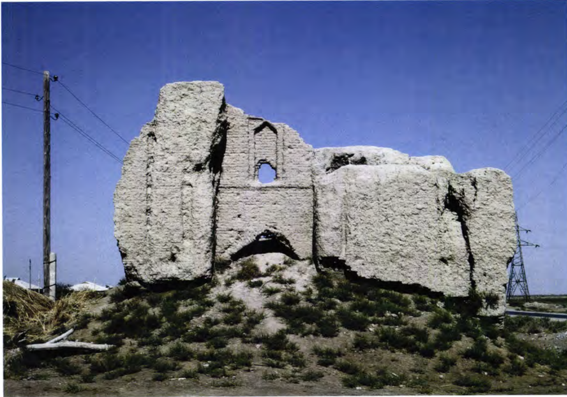
Figure 110 House east of Gyaur Kala [15]: the surviving section of the south façade. The central entrance consisted of an iwan with a doorway and 'overdoor' consisting of a rectangular panel and niche with stepped head. The walls were probably plain rather than corrugated or panelled.
