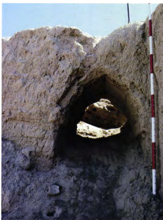
Figure 188 Greater Nagym Kala [2]: a doorway with a pointed head and bricks laid tile-wise; cf Kharoba Koshuk [25] (see Figure 287).
