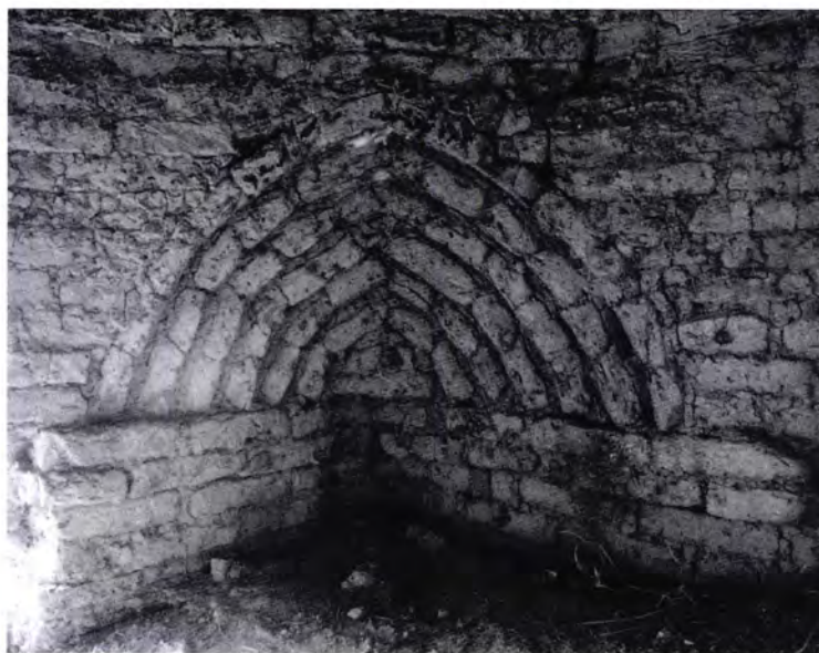
Figure 209 Garam Köshk [6]: the cone-shaped squinch formed of six concentric arches in Room 5.
