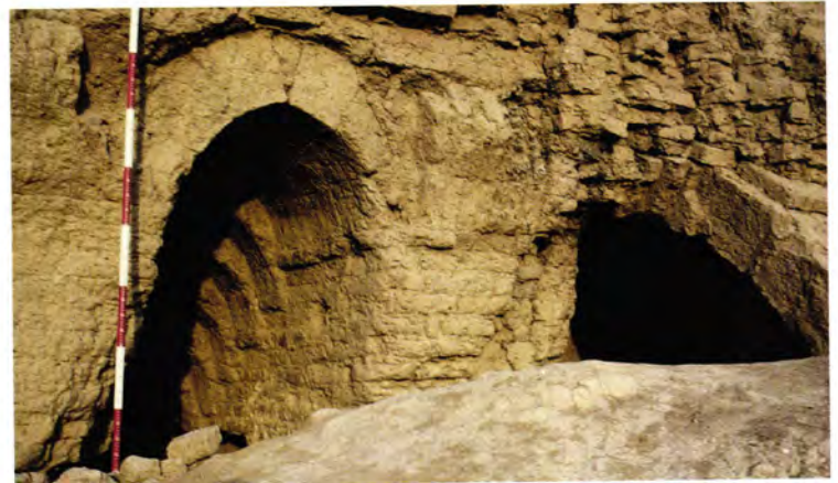
Figure 198 The Lesser Kyz Kala [4]: the bottom flight of the stairway (see Figure 197), covered with a stepped tunnel vault, and Room 6.
