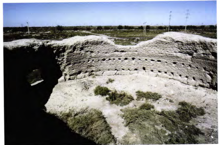
Figure 302 The interior of Ice-house 3 [29] looking north. The entrance (see Figure 303) is on the left. Note the numerous beam-slots.
