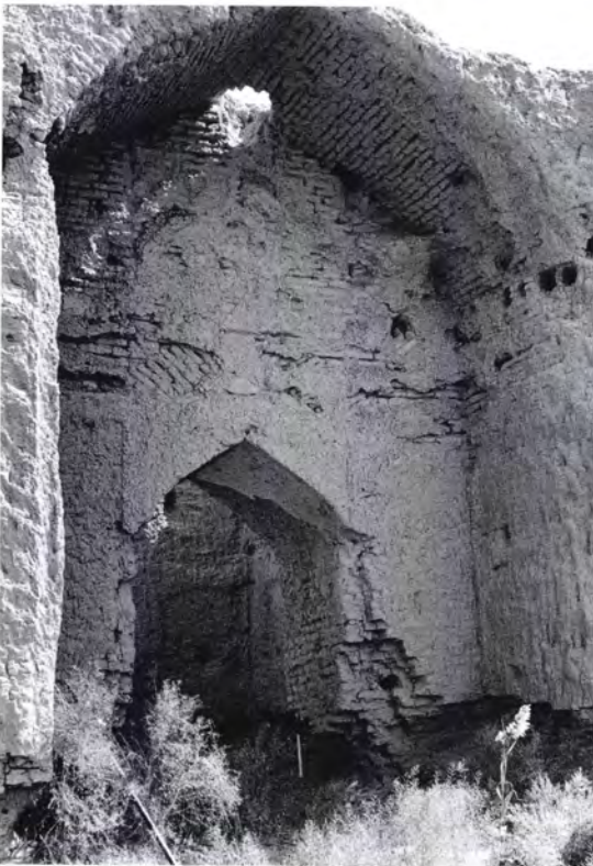
Figure 290 The iwan of the Timurid pavilion or Köshk Imaret [26]: traces of plaster survive over the original brickwork.
