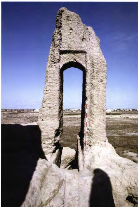
Figure 246 Porsoy Köshk [16]: the doorway of a tall, narrow, corridor-like room, 8, supporting the side walls of the north-east belvedere.
