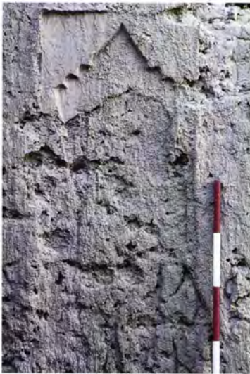
Figure 78 One of the narrow plastered panels with scalloped corners from the interior of the Kōshk Imaret [26], almost identical to that of the Abdullah Khan Kala palace (Figure 75): the plaster still retains traces of pink paint.
