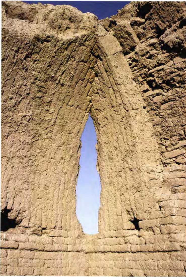
Figure 52 Another form of vault was the quadripartite lanceolate vault, seen here in Room 5 of the Greater Kyz Kala [1], where all walls curve inwards.
