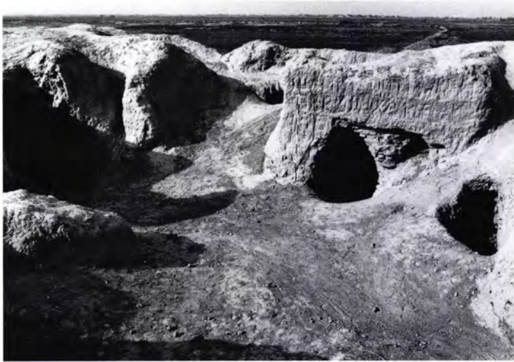
Figure 210 Garam Köshk [6]: view of the fragmentary remains of the upper storey looking west.
