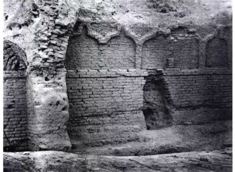
Figure 182 Part of Room 3 and Room 4 photographed by Cohn-Wiener in 1920 when more of the appliqué design above the string course survived.
