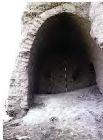
Figure 102 The high vaulted room, 3, in the exposed west corner of Garam Köshk [6].
