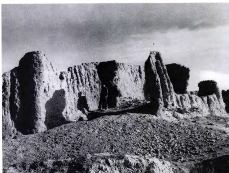
Figure 280 The remains of the west side and the interior of the 'Seljuk House', prior to the YuTAKE excavations. The course of fired bricks running along the west wall probably formed the base of the panelled decoration seen on the east side (see Figure 89). Note the slots for timber reinforcing beams.
