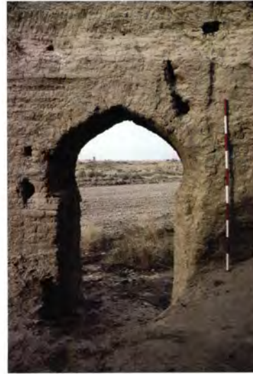
Figure 66 A four-centred doorway with re-entrants, a typical Islamic form, but only surviving at Merv in the elegant pavilion at Kurtly [21].
