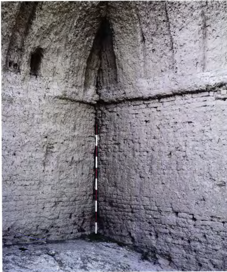
Figure 112 An unusual form of vaulting was employed on both tall rooms and low ones at Yakkiper Köshk [17]. The quadripartite lanceolate vault of Room 5 was reinforced or decorated with raised ribs or armatures.
