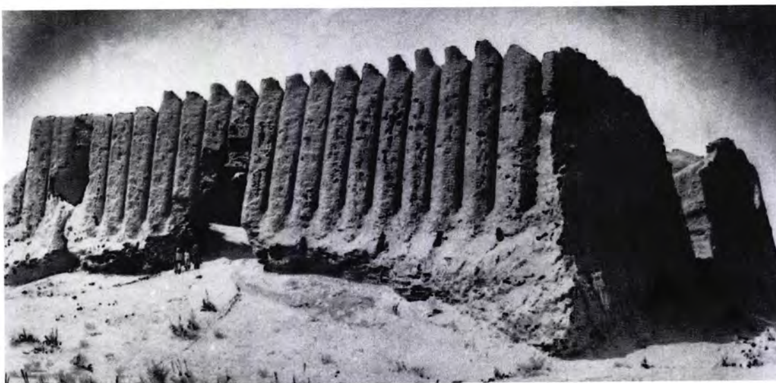
Figure 63 The principal, east façade of the Greater Kyz Kala [1], photographed by Zhukovsky in 1890 (1894, 165, fig 25) before the collapse of the central section. The arched opening in the centre of the upper storey would have been accessed by a ramp. The pointed form of the corrugations, forming a parapet around the flat roof, are well preserved.
