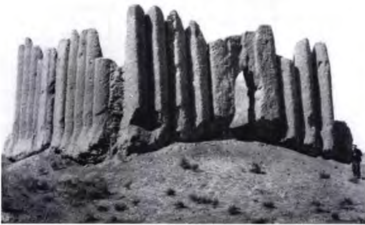
Figure 82 The köshk near Kelte Minar [13] in 1956, before the arched entrance collapsed (from Pugachenkova 1963, fig 5). In this köshk the corrugations encase the building but start nearer the ground than in the Group I–III köshks : this change probably reflects the increasing importance of rooms on the ground floor. There are flattened pilasters in the centres of the sides, flanking the entrance and either a very narrow entrance or a window.
