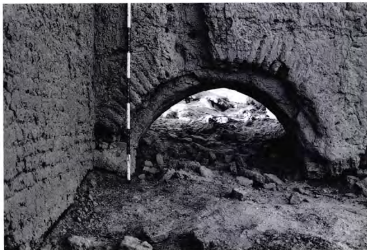
Figure 266 The palace in Shahryar Ark [20]: the doorway from Room 26 to Room 22 (see Figure 265) with bricks set radially on a course set tile-wise.
