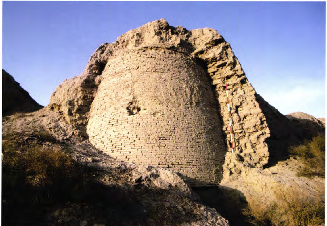
Figure 31 The two phases of construction of a tower belonging to the medieval walls of Sultan Kala.
