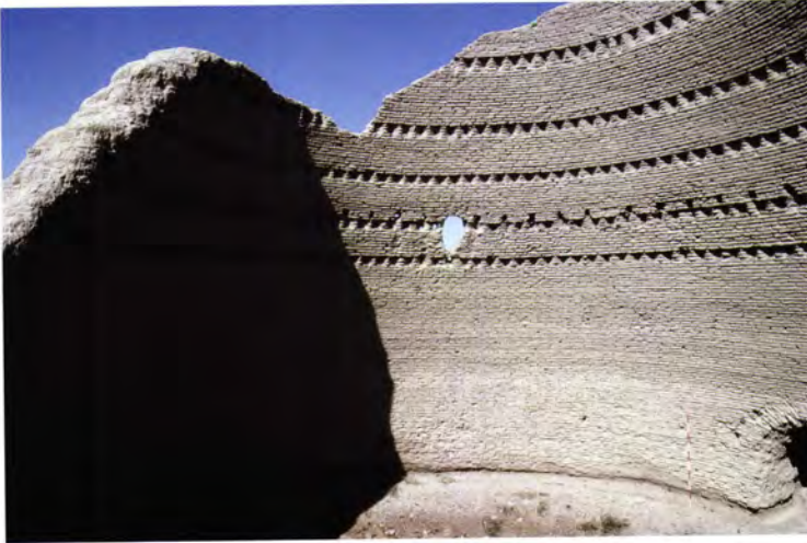
Figure 300 The interior of Ice-house 2 [28] with the north door on the right. Courses of diagonal brickwork embellish the upper zone.
