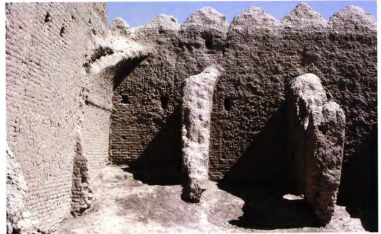
Figure 53 Much more modest barrel-vaulted rooms, 9 and 10, from the Greater Kyz Kala [1].
