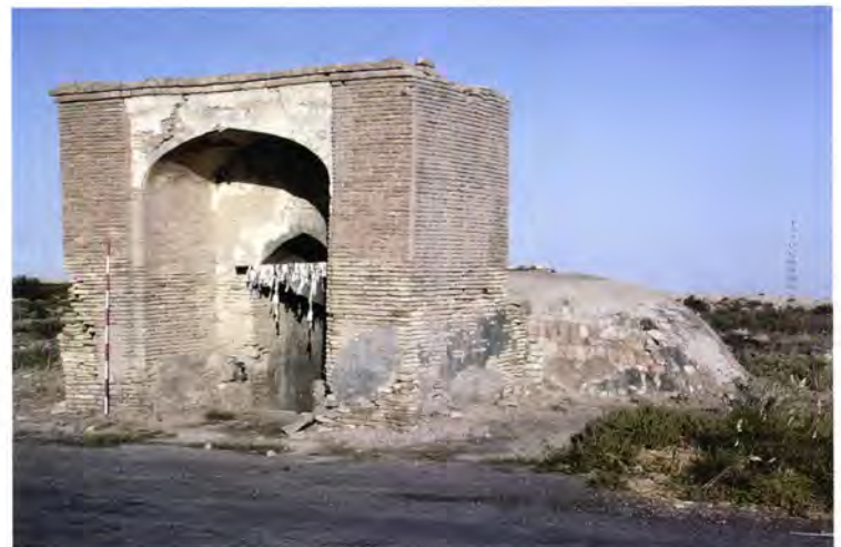
Figure 125 The sardoba forming part of the complex around the Timurid iwans or Askhab in the 1950s: this sardoba is still in use (YuTAKE archive). See also Figure 26.
