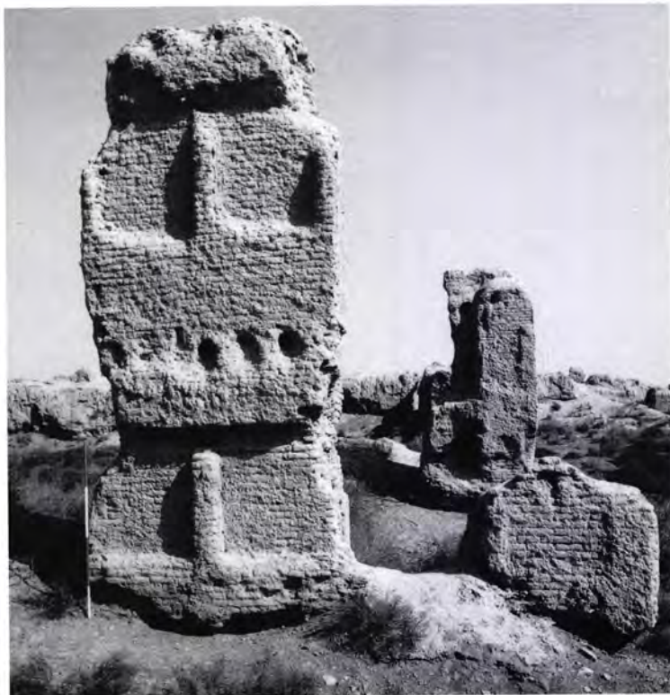
Figure 76 The frames of some panels in the Abdullah Khan Kala palace were formed of small, engaged columns (see also Figure 24).
