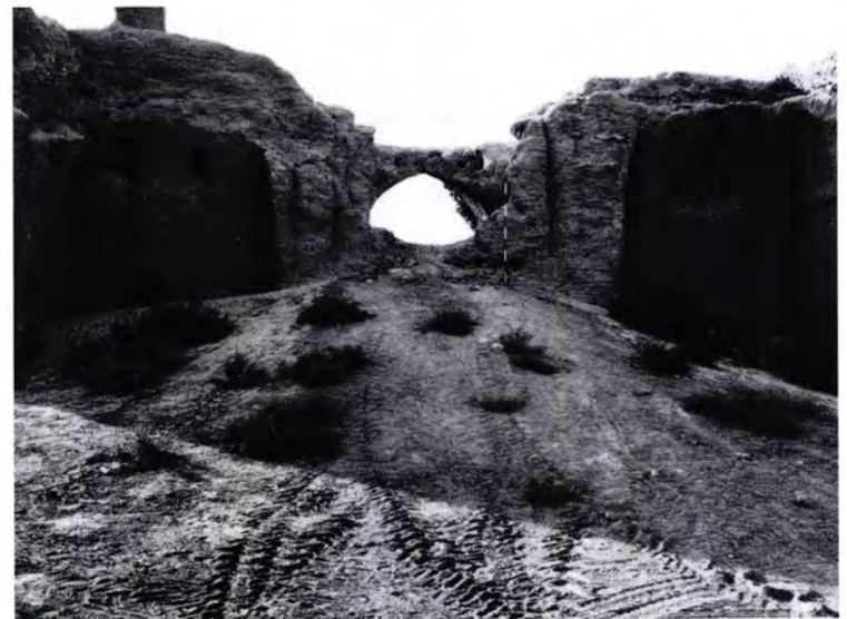
Figure 252 The tall Rooms 3 to 5 revealed by the collapse of the north-west façade of Yakkiper Köshk [17]. They were roofed
