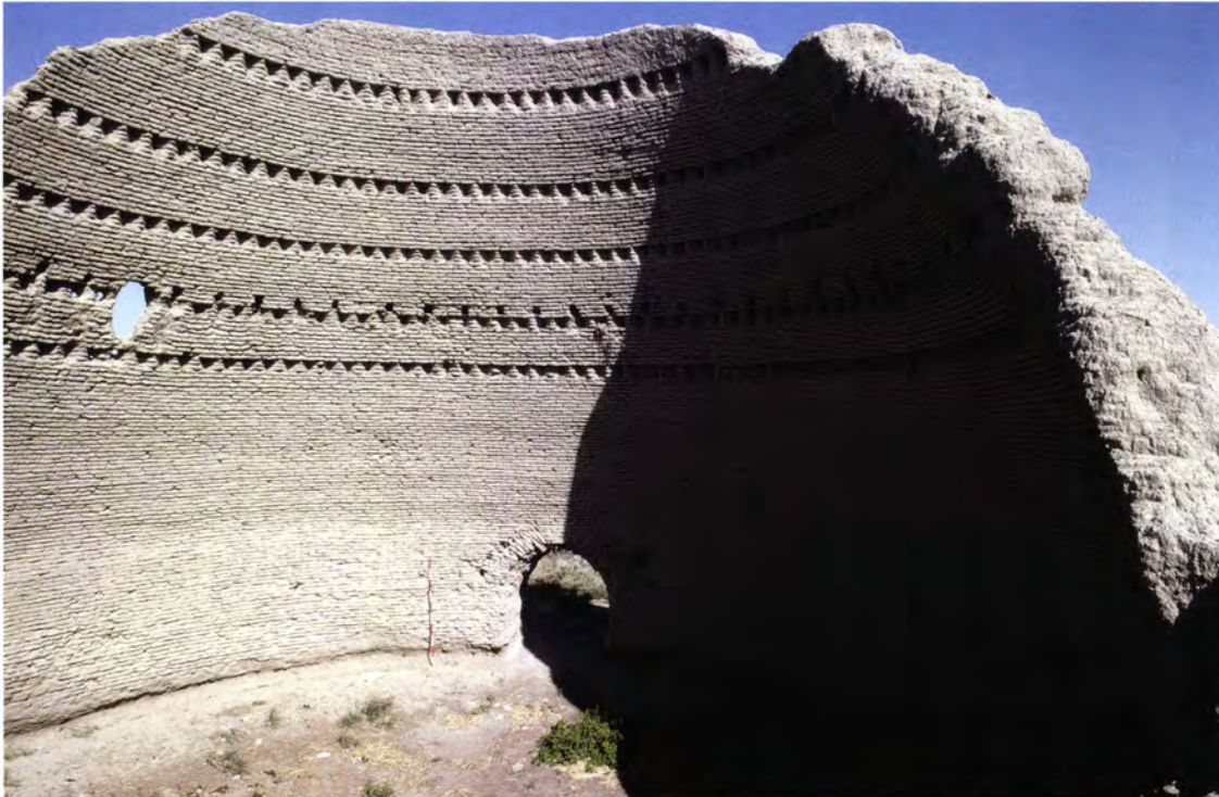
Figure 49 The great corbelled dome of Ice-house 2 [28], relieved by bands of decorative brickwork. The entrance was in the north; there were also two deep niches.
