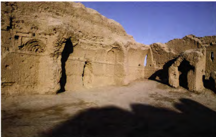
Figure 181 Rooms 3 to 5 and the stairway in the north-west corner of the Greater Kyz Kala [1]. Note the variety of roofing employed, the cone-shaped squinch in Room 3 and the quadripartite elliptical vaults in Rooms 4 and 5, that of Room 4 being embellished with an appliqué design above the string course.
