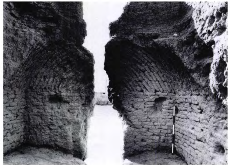
Figure 315 The 'school ding ' [32f] in the Kalinin kolkhoz playground: the barrel vault is closed with a semicircle of bricks (see Figure 314).
