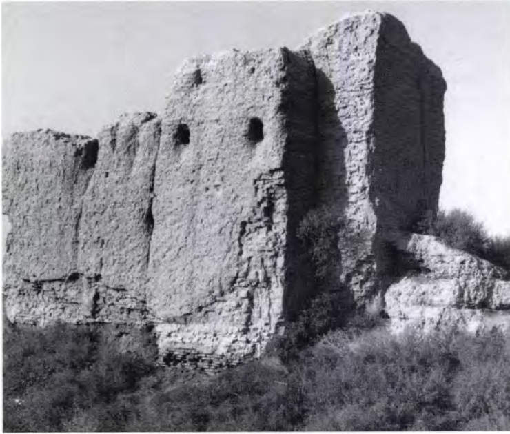
Figure 237 House east of Gyaur Kala [15]: the surviving section of the east façade, with the arch of the central iwan rising on the right. Note the slots for timber reinforcing beams.
