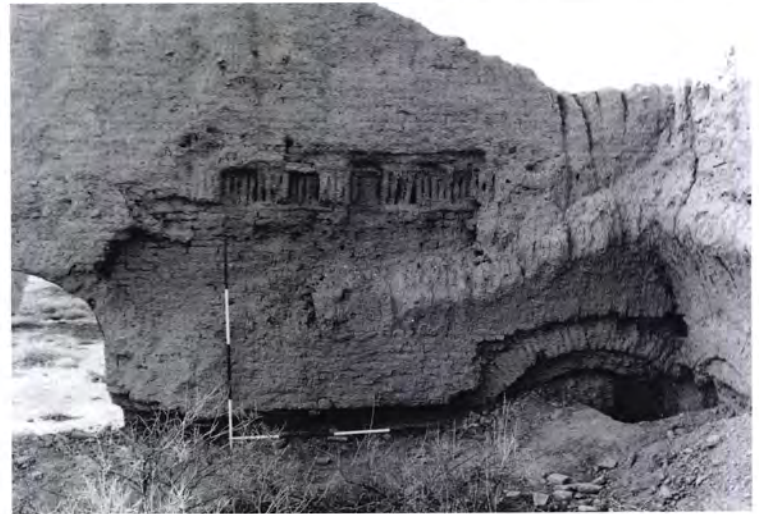
Figure 264 The palace in Shahryar Ark [20]: a small 'landing', 9, covered with a low quadrupartite vault. The arches of the stairway are formed of bricks set radially.
