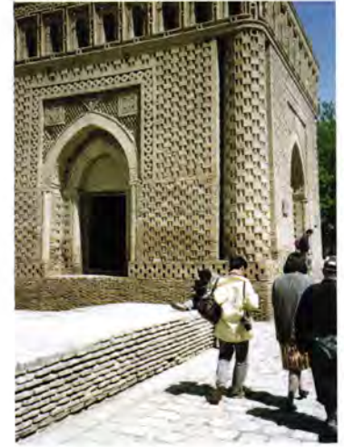
Figure 70 The fashion for decorative brickwork reached its height at the earlier Samanid mausoleum in Bukhara.
