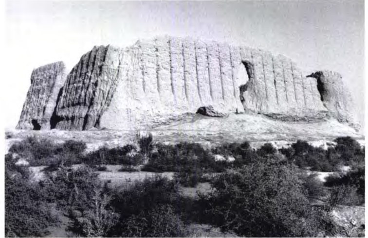
Figure 178 The eroded north and west façades of the Greater Kyz Kala [1] from the north west. Runnels indicate the original location of the corrugations.
