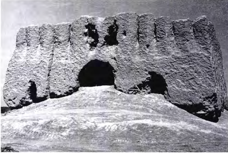
Figure 99 The south-east façade of Garam Köshk [6] in the 1980s with access at ground level via a central iwan. The side openings are enlarged window slots.
