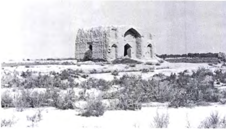
Figure 288 The façade and north side of the Timurid pavilion or Köshk Imaret [26] in 1961, photographed by S Chmelniczki.
