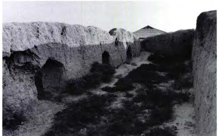
Figure 306 The interior of the better-preserved southern room of the nineteenth-century merchant's house [31]. It was roofed by cross vaults and balkhi vaults.
