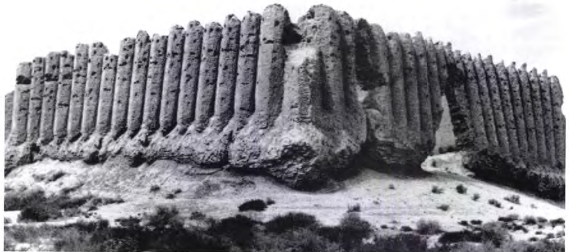
Figure 95 The south and east façades of Greater Kyz Kala [1] photographed in 1971 (Atagaryev and Pilyavsky 1974, 117) before the arch of the entrance on the east collapsed.
