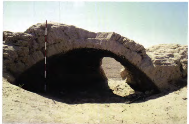
Figure 222 Penapir Köshk [9]: view of the surviving dome of Room 4 in 1997. The interior was covered by an exceptionally strong clay and straw mortar, blackened by smoke. Part of it had collapsed by 1998.
