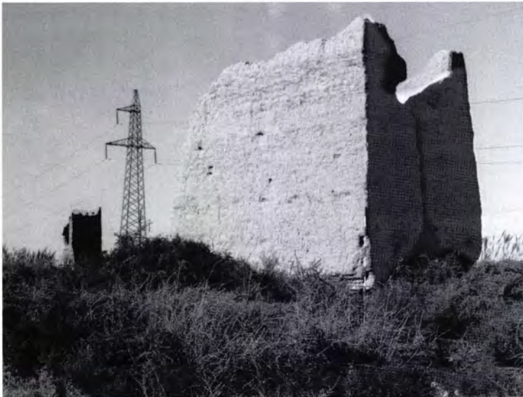
Figure 309 Electricity Station Dings 2 [32b] and 3 [32c] (see Figures 310 and 311) from the south.
