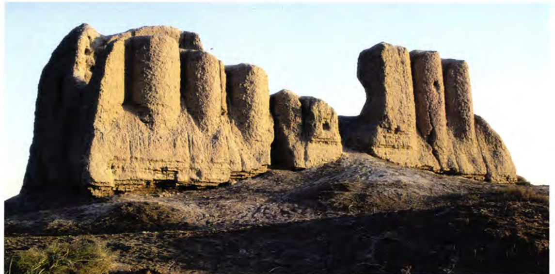
Figure 100 The south façade of the Lesser Kyz Kala [4]. The centre of the façade is occupied by a raised rectangular panel, framed by half-corrugations.
