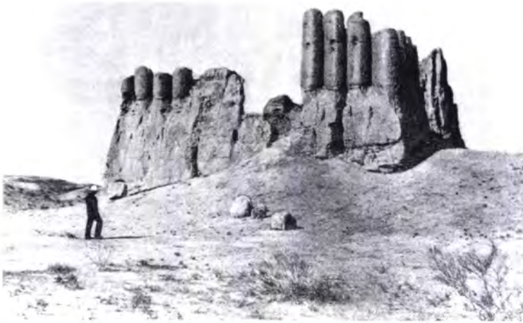
Figure 103 The south and east façades of Suli Köshk [7] in the 1950s (Pugachenkova, 1958, 156). Note how the corrugations start much more abruptly than those of the preceding Group I and II köshks.
