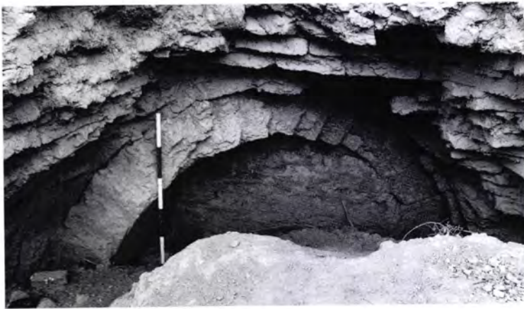
Figure 196 The Lesser Kyz Kala [4]: the barrel vault of Room 3 behind the south façade on the lower storey. Note the floor of the upper storey.
