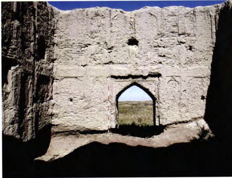
Figure 292 The interior of the Timurid pavilion or Köshk Imaret [26], with registers of plaster panels, alternately wide and narrow.
