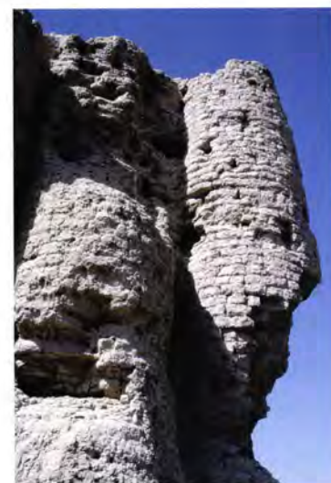
Figure 106 Note the curved bricks of the corrugations of Lesser Nagym Kala [11], and the deep slots left by the timber tie-beams.
