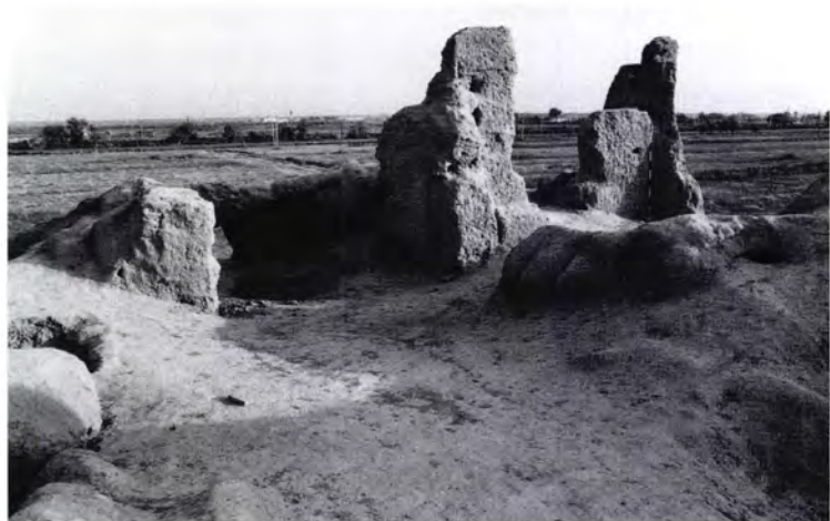
Figure 217 Suli Köshk [7]: the northern and central area of the upper storey. The stairway was on the left, the top of the domed room, 2, in the centre,
