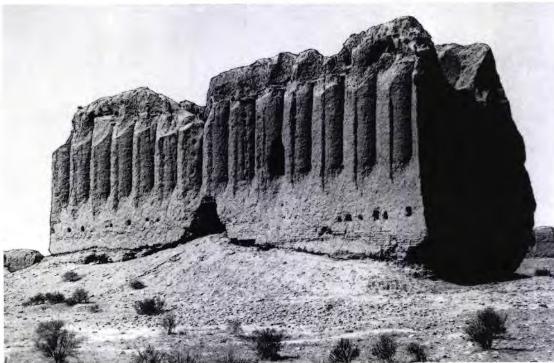
Figure 119 The kepter khana in Shahryar Ark [22] from the north east, photographed by Zhukovsky in the 1890s (1894, 121). Note the well-preserved corrugations with a central rib, the remains of the row of squinch arches above the corrugations, the small entrance at ground level and the beam-slots in the plain skirt.
