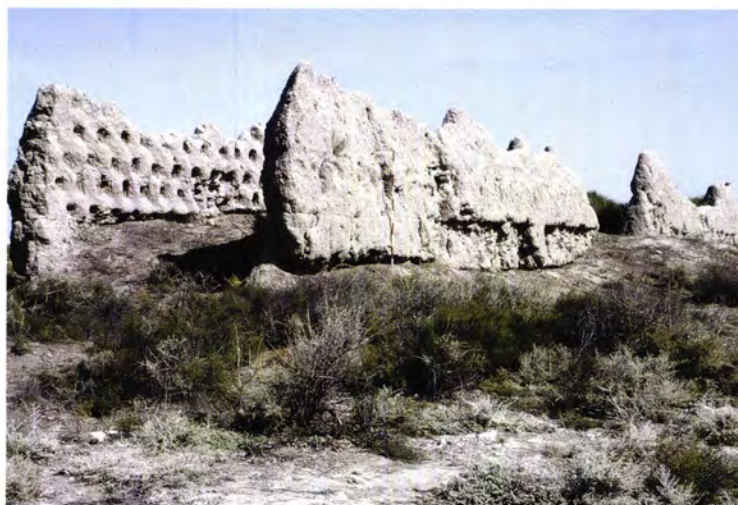
Figure 282 The kepter khana [24] in Iskandar Kala from the north east, showing the northern façade and part of the interior with serried ranks of hooded niches along the southern wall (see also Figure 121).
