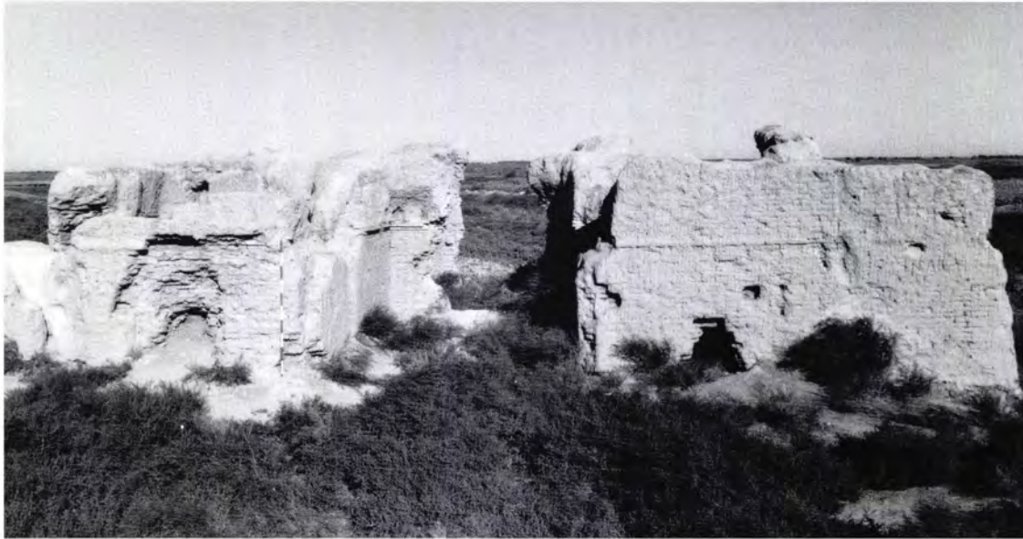
Figure 271 The pavilion at Kurtly [21]: the north-east façade opening on to the platform. The iwan was vaulted and ended in a semi-dome, which rose from elaborate squinches with a trilobate motif in the centre on a fired-brick string course.
