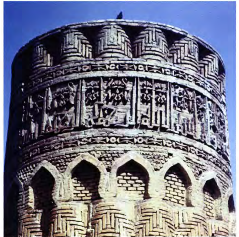
Figure 83 The minaret at Dzhar-kurgan in the Surkhan Darya valley near Termez, dated to 1108–9, is decorated with corrugations terminating in a row of squinch arches.
