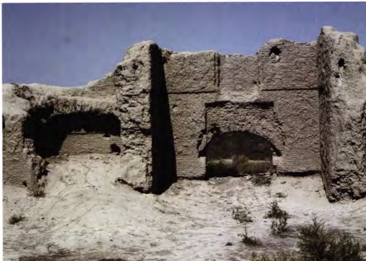
Figure 68 The wide doorway with a segmental arch in the north iwan of the palace in Shahryar Ark [20]. Note the raised panels above.
