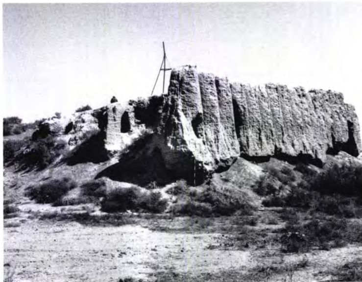
Figure 185 The collapsed west and south façades of Greater Nagym Kala [2]. The doorway with a pointed head (see Figure 188) can be seen in the centre.
