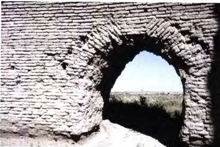
Figure 127 The north doorway of Ice-house 2 [28] from the interior. The 'keystone' is formed of horizontal courses of brickwork.
