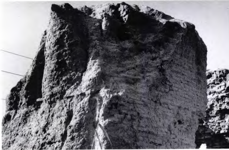
Figure 225 The köshk [10] south of Gyaur Kala: detail of the west side of the south façade showing at the upper right a few vertical bricks belonging to the springing of the central iwan.
