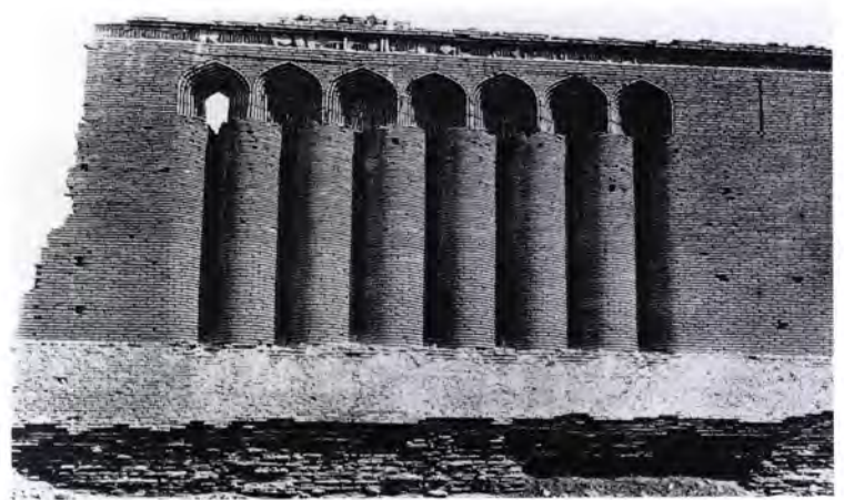
Figure 80 The corrugations of the Seljuk caravanserai at Rabat-i Malik (1078) are used in panels instead of encasing the building and are ‘short’, rising abruptly from the plain skirt of the building and
