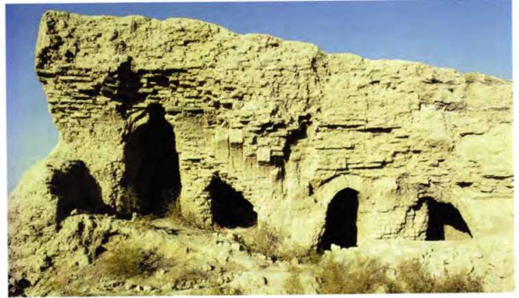
Figure 197 The Lesser Kyz Kala [4]: the stairway in the south-east corner, revealed by the collapse of the east façade in 1991. There were three flights, with rooms accessed from the landings. Only the springing survives of the central flight.
