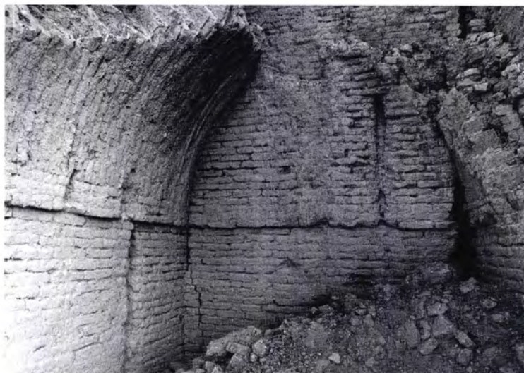
Figure 247 Porsoy Köshk [16]: Room 6. The barrel vault rises from a three-brick string course.
