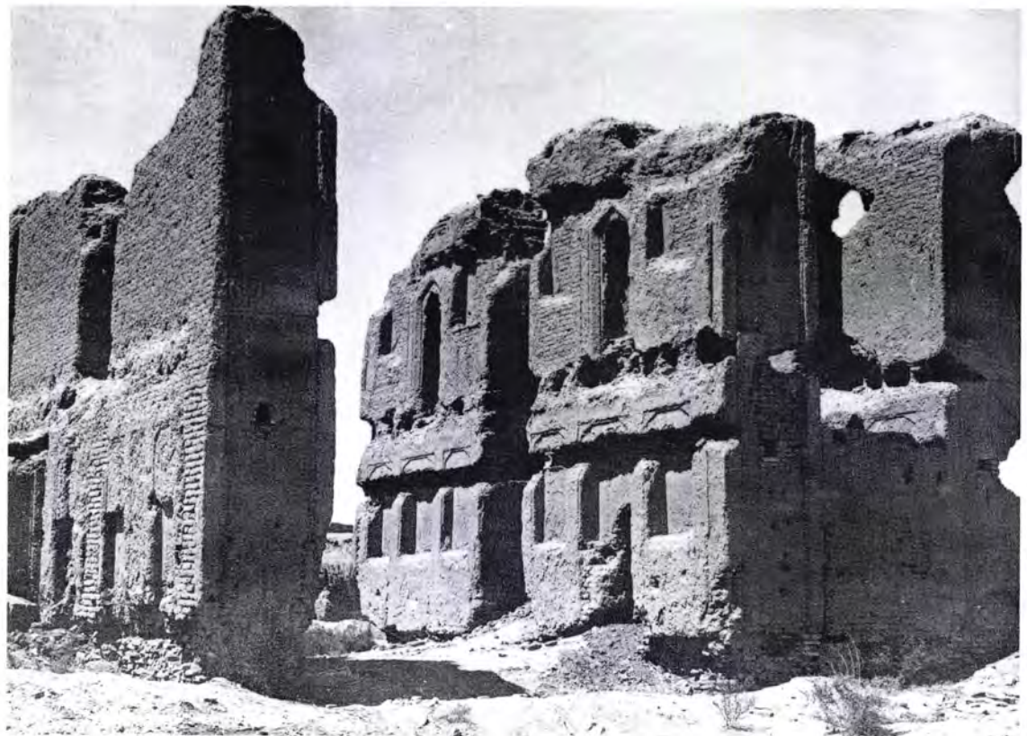
Figure 24 Part of the palace in the post-medieval citadel in 1890, photographed by Zhukovsky. Note the doorways, the beam-slots for the timber floors and the panels of plastered decoration.
