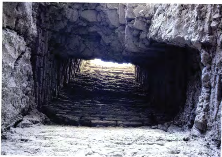
Figure 297 One of the ventilation chimneys of Ice-house 1 [27].
