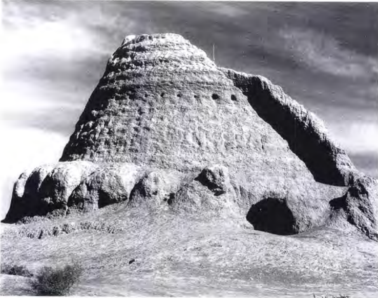
Figure 126 Ice-house 2 [28] in 1954: the western niche has been opened to allow access and part of the dome has collapsed (YuTAKE archive).
