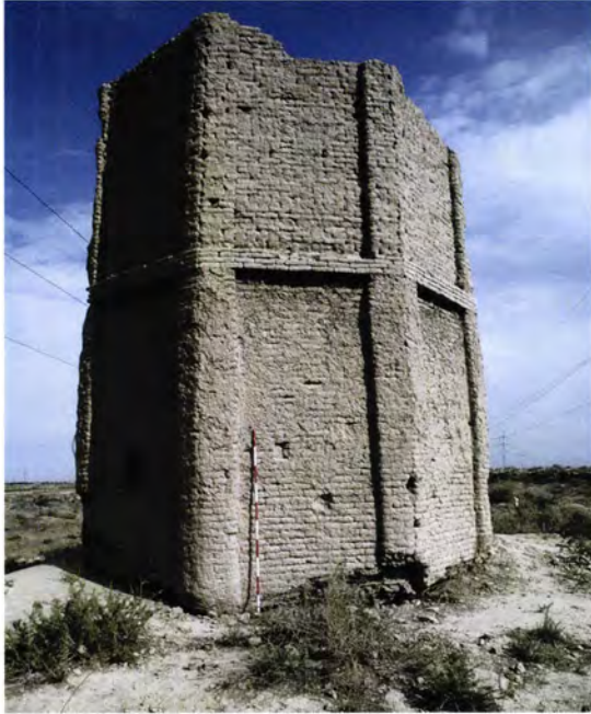
Figure 308 Electricity Station Ding 1 [32a], the only octagonal ding surviving in the oasis, and the only one with decorated external walls. There is no access to the ground floor: the upper storey would have been reached by ladder.
