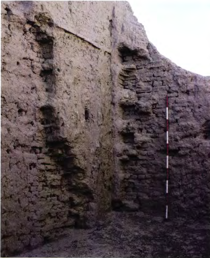
Figure 120 The interior of the kepter khana in Shahryar Ark [22]. This long, narrow room was roofed with transverse vaults carried on pilasters, the vault rising from a course of fired bricks at the top. Panels of deep niches arranged in a chequerboard pattern occupied the end walls and the spaces between the pilasters.
