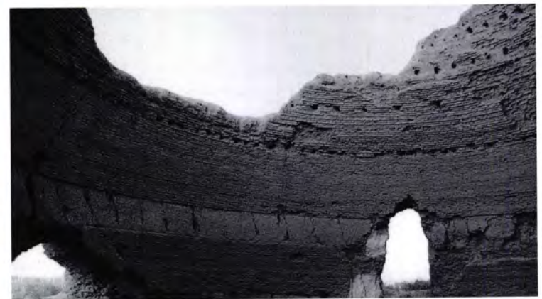
Figure 294 The circular interior of Ice-house 1 [27]: the remains of the north door are on the left, and a broken chimney can be seen towards the right. The niche has been destroyed. The lower parts
