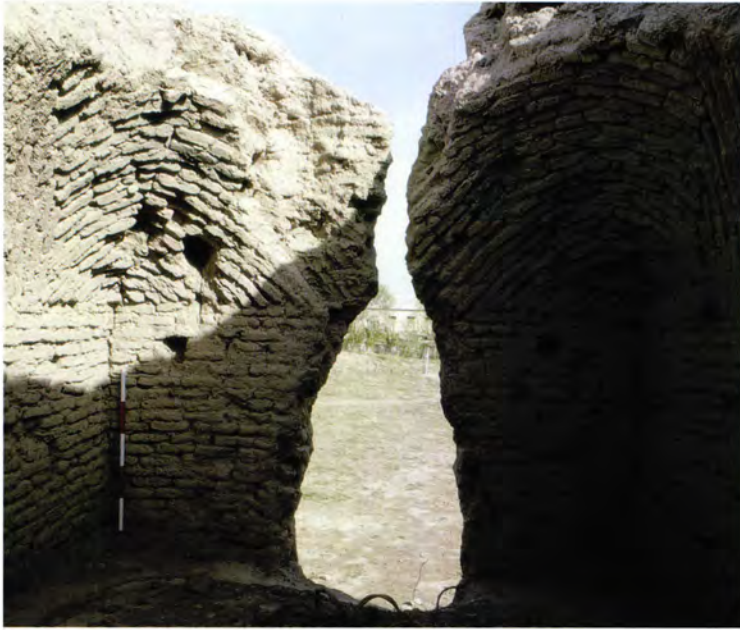
Figure 314 The 'school ding ' [32f] in the Kalinin kolkhoz playground is unusual in having different forms of vaulting at each end, in this case a squinch vault.
