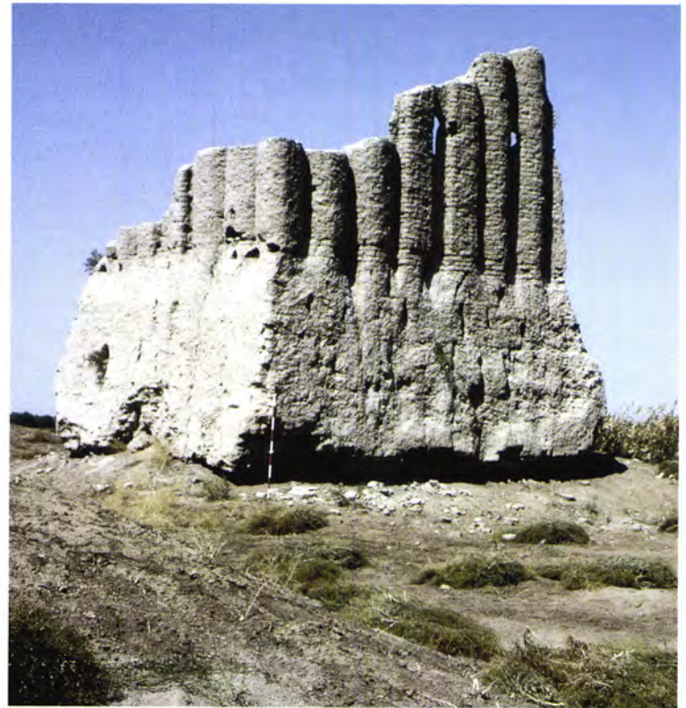
Figure 229 The south-east corner of Durnali Köshk/ Ding . The two central 'corrugations' on each side have been flattened and widened to form pilasters, separated by a slightly wider recess than usual to allow for windows (cf Kelte Minar, Figure 233). Note the slots for timber reinforcing beams. The tower formed part of a walled complex of buildings.
