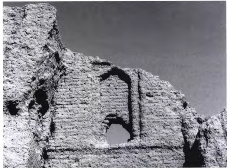
Figure 238 The left arch of the iwan of the House east of Gyaur Kala [15], with a rectangular panel with a stepped arched niche above the doorway, similar to those at Ovliali Köshk [14] and above the doorways of the central room of Porsoy Köshk [16].
