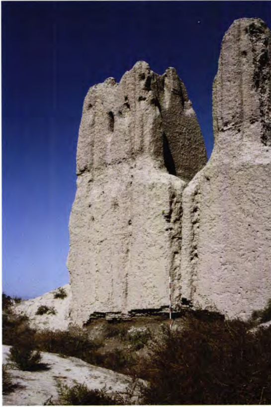
Figure 243 Porsoy Köshk [16]: the only surviving section of external wall is on the south east. Traces can be seen of the decoration of the élite upper storey with engaged ribbed pilasters, framing the central opening of the belvedere (see Figure 111).
