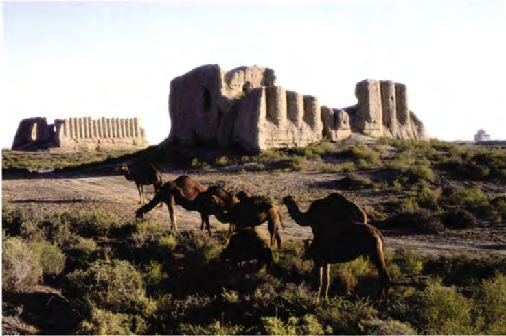
Figure 177 The Lesser and Greater Kyz Kalas, [4] and [1], from the south west; the Mausoleum of Sultan Sanjar is in the distance.
