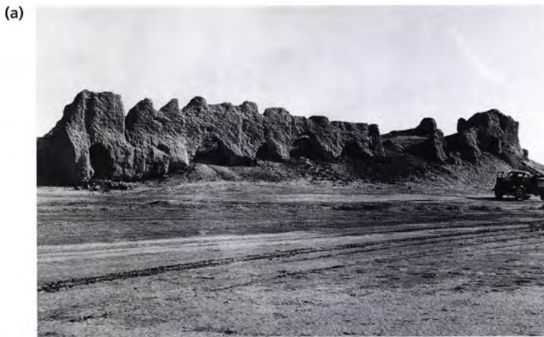
Figure 284 The south façade of Kharoba Koshuk [25] in 1966 (a) and 1981 (b). There has been considerable deterioration since that time.
