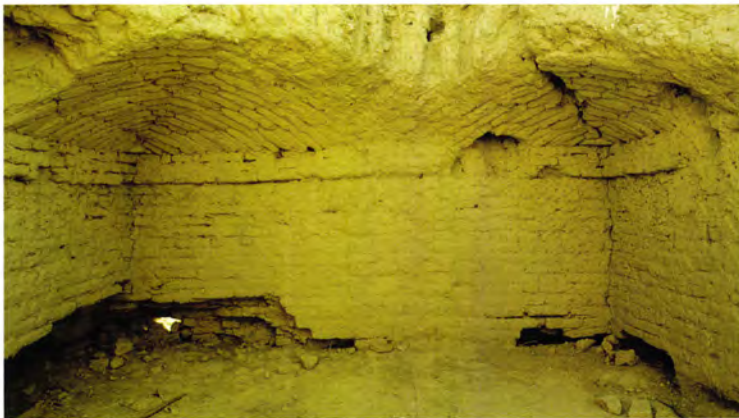
Figure 50 The squinch or balkhi vault was employed at Merv when a low domed room was required, as in
