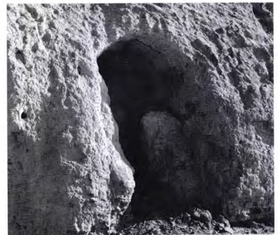
Figure 287 Kharoba Koshuk [25] in 1966: a doorway in the south façade with the arch formed of bricks set tile-wise, as in the Greater Nagym Kala [2] (see Figure 188).
