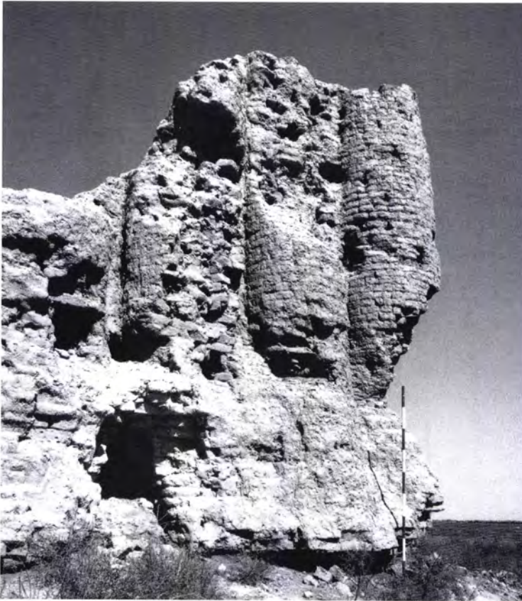
Figure 228 The Lesser Nagym Kala [11]: detail of Figure 226. The corrugations are formed of curved bricks and rise from a course of fired bricks.
