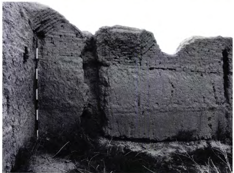
Figure 307 The cross vaults and balkhi vaults seen at the south-west end of Figure 306.
