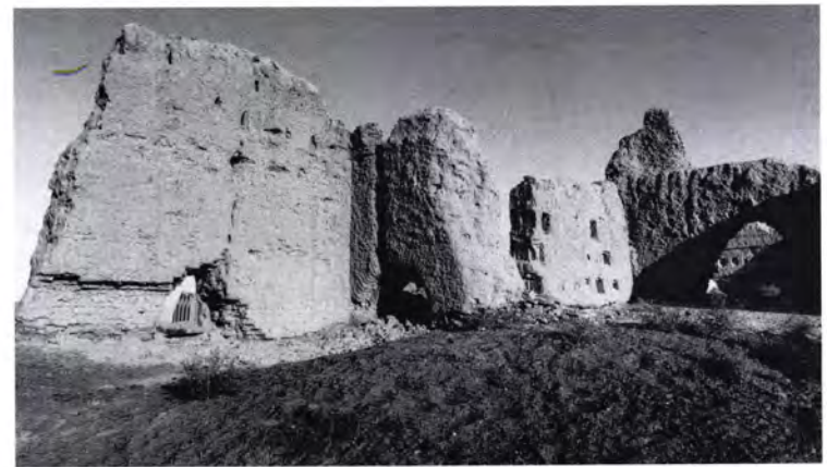
Figure 265 The surviving west walls of Rooms 23 and 26 in the south east of the palace in Shahryar Ark [20]. The wall of Room 26
