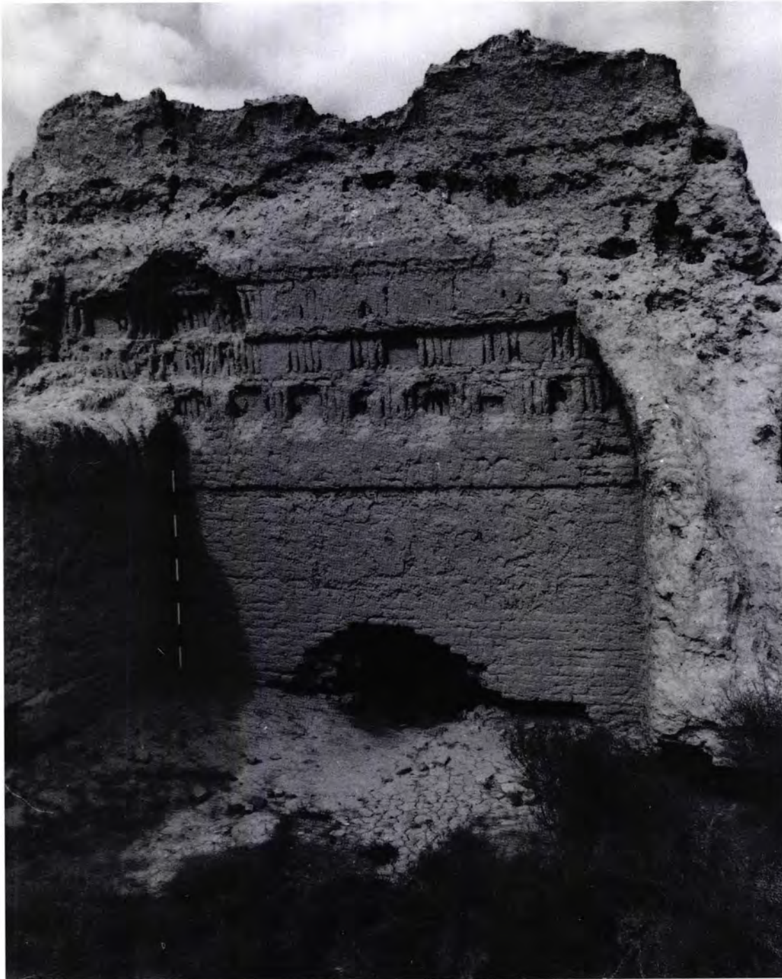
Figure 37 Chequerboard brickwork set on a brick string course, presumably employed to decorate the upper back wall of Room 17 in the Ark palace [20], as well as continuing behind the vault.
