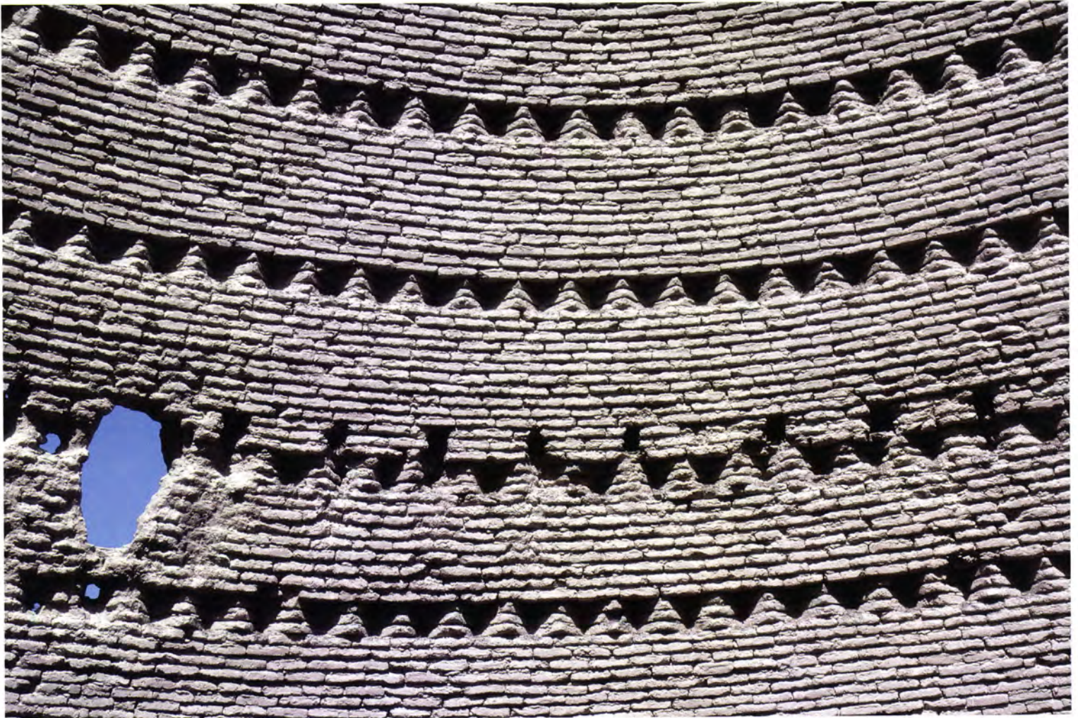
Figure 114 The interior of the great cone of Ice-house 2 [28] with its rows of diagonally set bricks.
