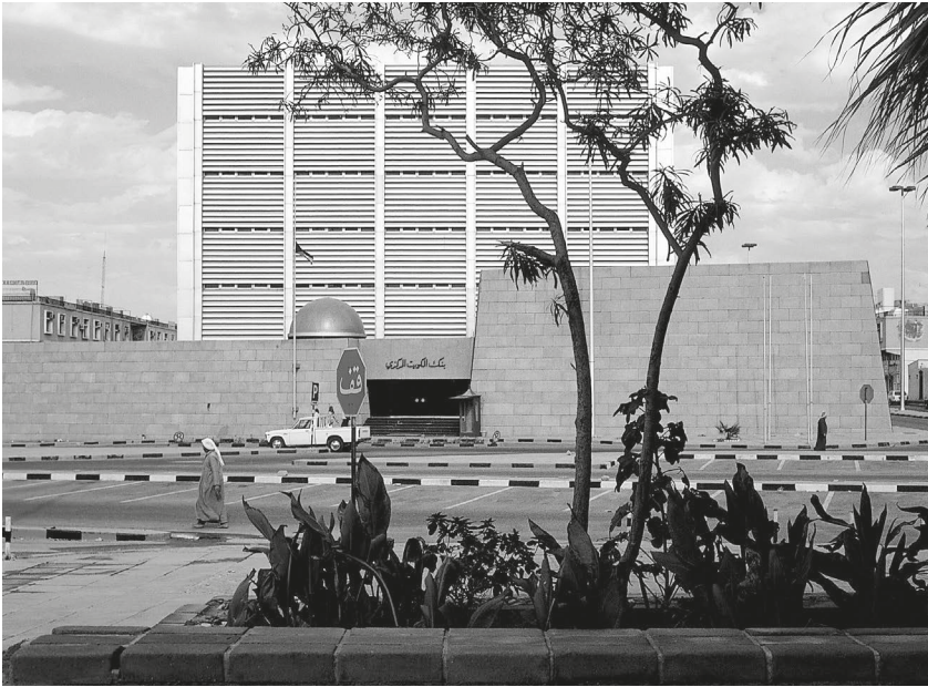
Central Bank of Kuwait, prior to renovation. The building was design by Arne Jacobsen in 1966 and constructed by Dissing+Weitling from 1973 to 1976 (Source: Dissing+Weitling. Reuse not permitted).
