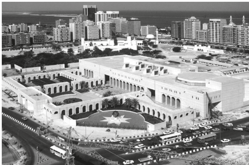
fig.1 The Architects Collaborative, Cultural Foundation – Abu Dhabi National Library and Cultural Centre, 1974–1979, and Qasr Al-Hosn at upper left (Source: Aga Khan Trust for Culture, courtesy of the architect, 1985. Reuse not permitted).
