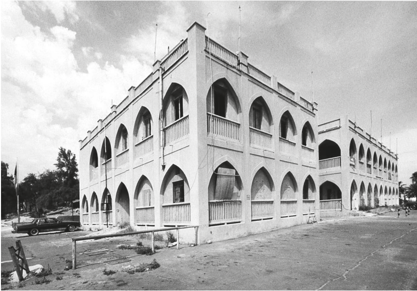
American Mission Hospital, locally known as Al-Amricani, before the renovation (Photo: Abdulkareem Al-Ghadban, 1993. Reuse not permitted).
