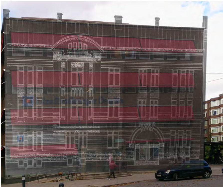
Fig. 8. The art nouveau style living quarters of Janse's candy factory at Handverkaregatan 51 (demolished in 1971) in an overlay montage with the present building on the same site.
