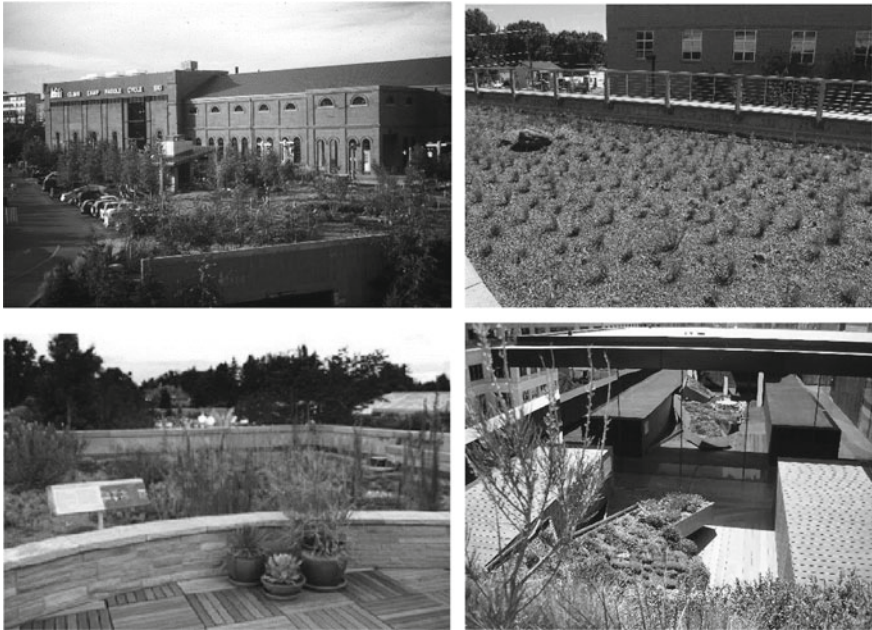
Fig. 11.22 Green roof technique in Denver, CO, USA, for stormwater management (Modified from: Agency 2017)
