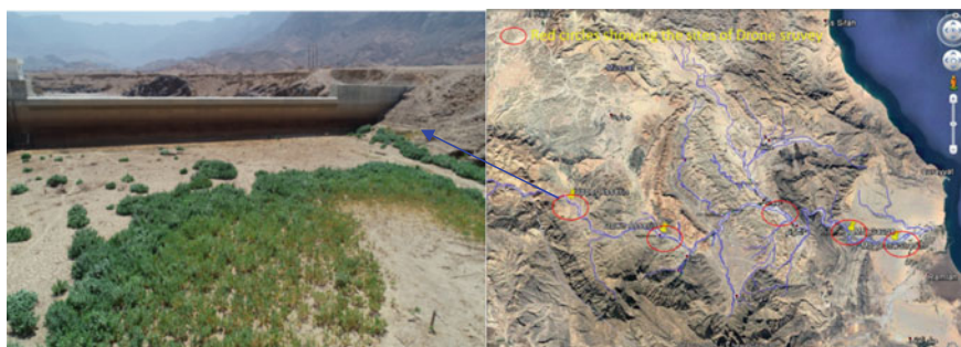
Fig. 15.16 Satellite image showing the sites for the drone survey of Wadi Mijlas, Oman, on the right and the drone photograph of Asserin Up Dam, Wadi Mijlas, Oman on the left
