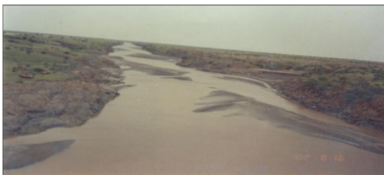
Fig. 18.11 Accumulation of silt downstream due to insufficient discharge in flush operations
