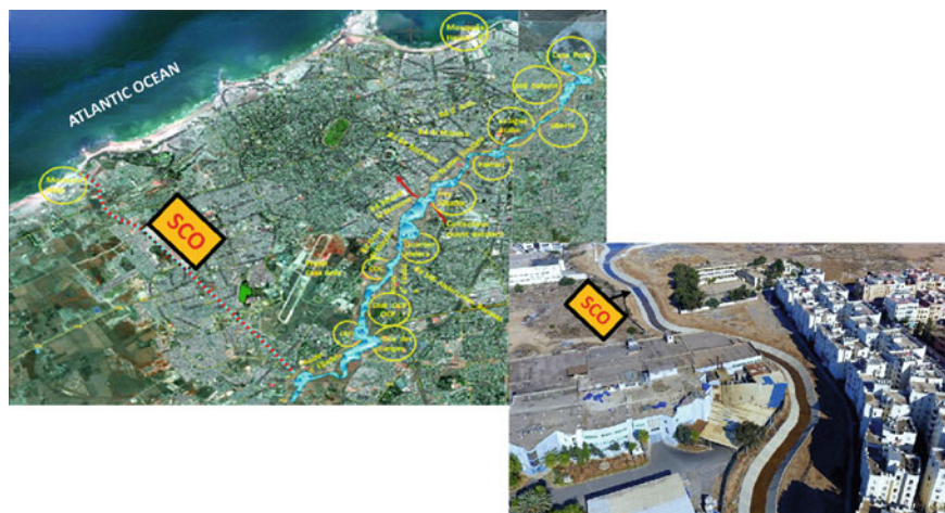
Fig. 2.19 Wadi Bouskoura channelization with the SCO drainage system for Casablanca flood control (Source LYDEC 2014; Casa Aménagement 2020)
