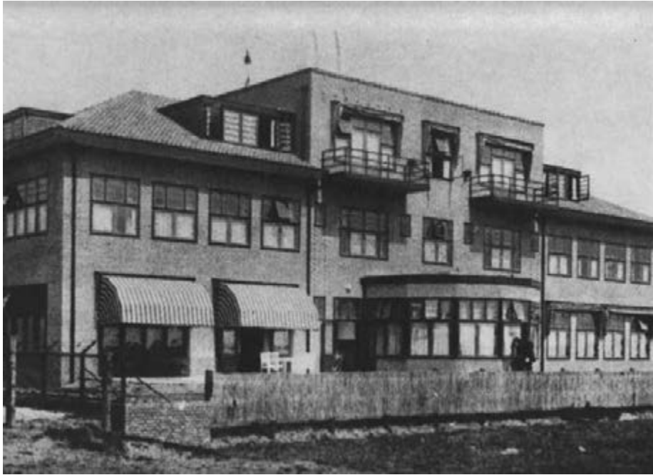
Figure 3.6: The backside of the building in 1929; photographed about a week after the inauguration in June 1929. On the left of the photo what is called the “right wing”, as seen standing in front of the building in Roodenburgerstraat. On the ground floor, left: the director’s offices under the striped awnings. On the second floor, left: the four windows of the small girls’ dormitory. On the third floor, centre: the windows of the two sickbays (with balconies) and in between the room of a nanny or nurse. Under the sloping roof: the two attics with the rooms for resident staff (with dormers).
