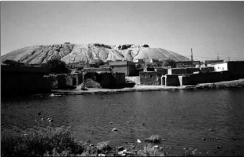
Figure 7.2. Rising groundwater due to heavy application of irrigation water forms “lakes” such as this in many villages in the southern part of the Harran plain, inundating houses and posing health risks from stagnant water. Photo by Leila M. Harris.
