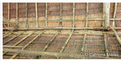
qötu gövr ~ roof beam
