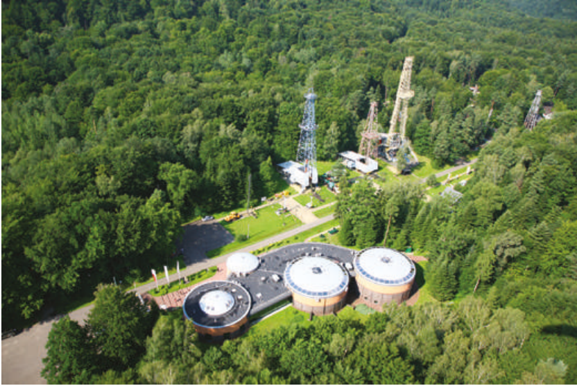
Figure 33: The antique oilfield in Bóbrka – contemporary view. Source: The Ignacy Łukasiewicz Oil and Gas Industry Museum in Bóbrka
