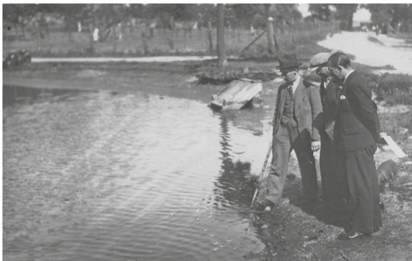
Figure 10: Leaking crude oil. Source: Subcarpathian Museum in Krosno
