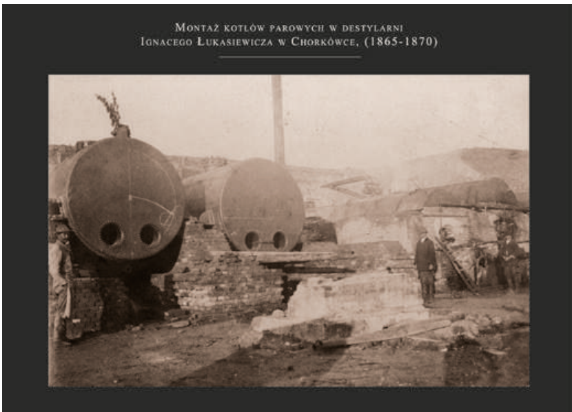
Figure 16: Installation of steam boilers at the distillery in Chorkowka. Source: Subcarpathian Museum in Krosno
