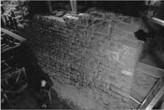
Fig. 7. Westside of the tower with angular ashlar masonry
