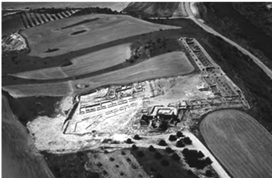
Fig. 2. The excavation from 1996
