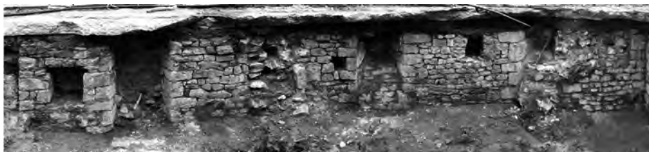
Fig. 12. Magdeburg – Breiter Weg-northern section, east side. In the course of sewer renovation works, cellar brickwork, probably of Romanesque origin, was unearthed immediately below the modern road level, excavated while accompanying the digging of a sewage canal in summer 2003
