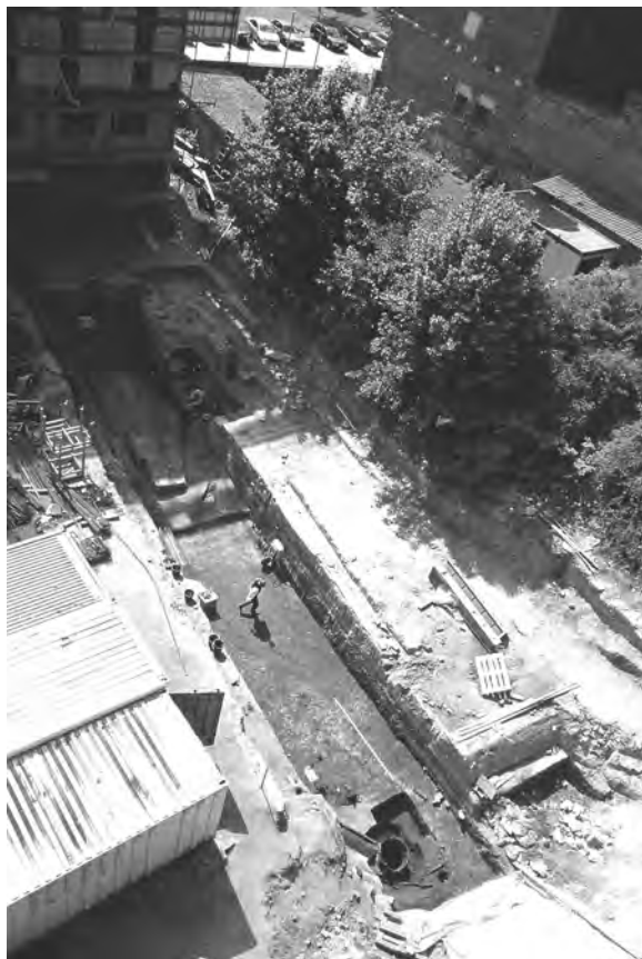
Fig. 9. Magdeburg – Große Klosterstraße/Fürstenwallstraße. View of the excavation trench from the north-west
