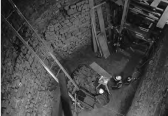
Fig. 9. Inside of the circular wall; from the west
