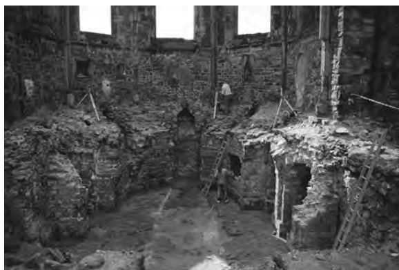
Fig. 7. Magdeburg – Johanniskirche. Romanesque crypt beneath the Gothic quire in the course of excavations before its reconstruction (twelfth century)
