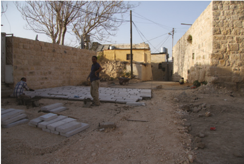
Fig. 4.3 Intervention of street paving. © Mutual Heritage 2009.
