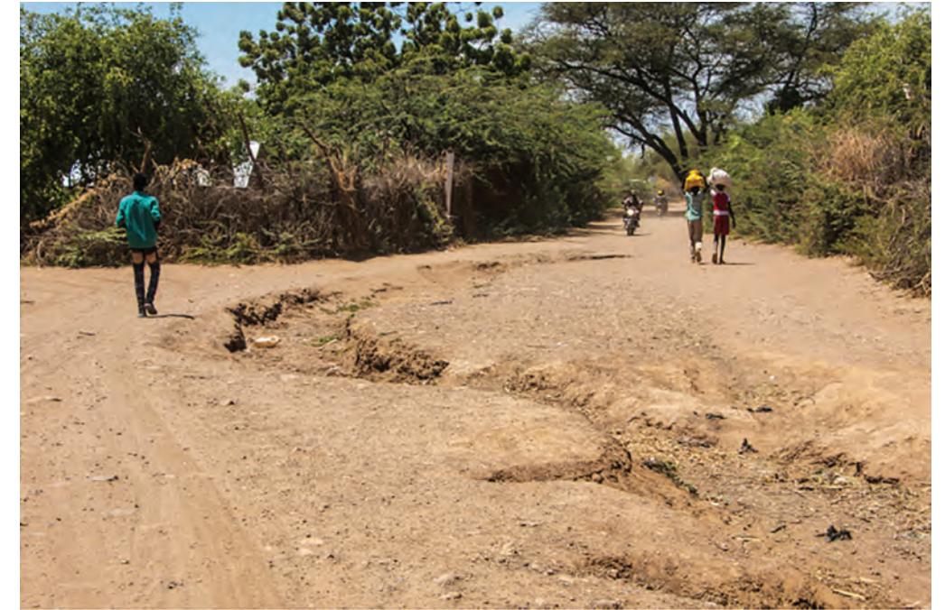
2.16 Kakuma refugee camp. Bottom left: Map of Kakuma showing the areas that flood during the rainy season. Top and bottom right: Photographs of the seasonal rivers/flood-prone areas called 'lagga' between Kakuma phases I and II. September 2016. © Amorós Elorduy.
