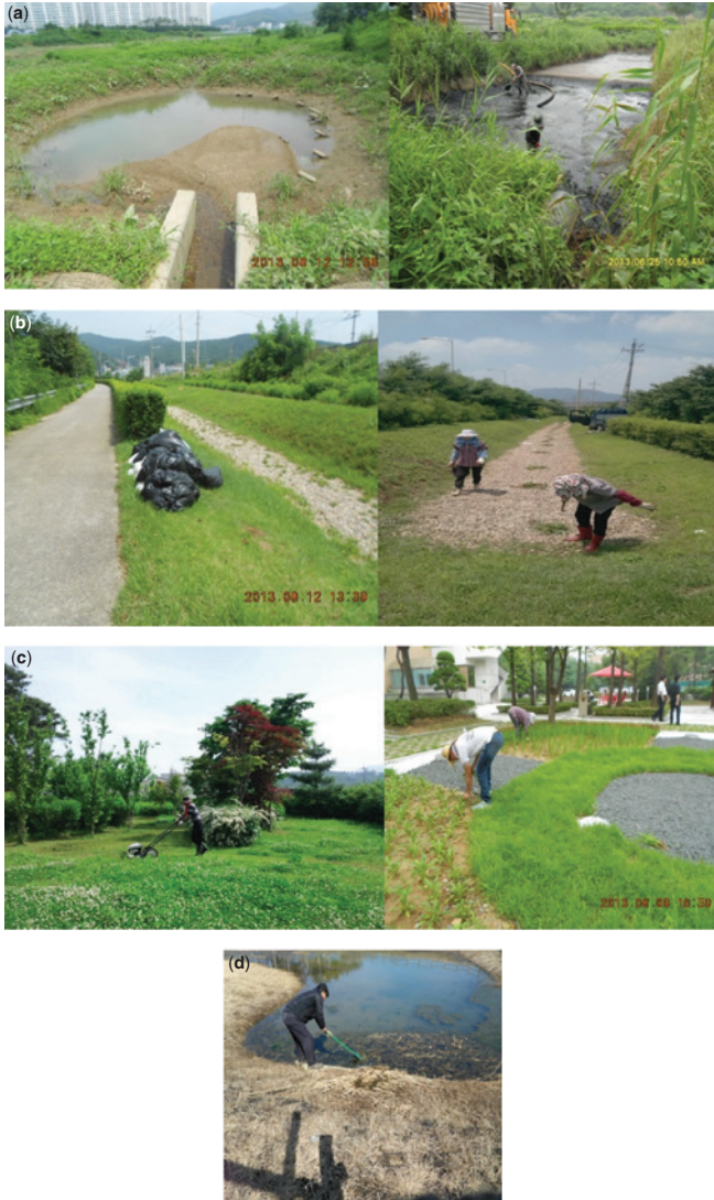
Figure 12.16 Some examples of maintenance activities four major rivers' BMP sites in South Korea. (a) Dredging for sediment removal, (b) Litter removal, (c) Gardening for plant removal and (d) Removal of dead plants
