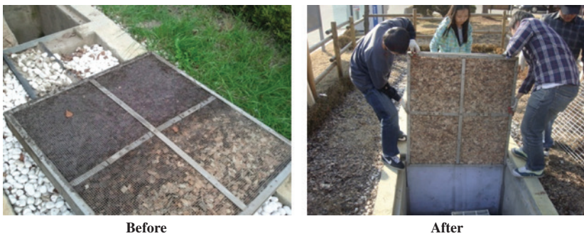
Figure 12.9 Woodchip in the vertical media cartridge was replaced as part of the non-routine maintenance in the infiltration trench.
