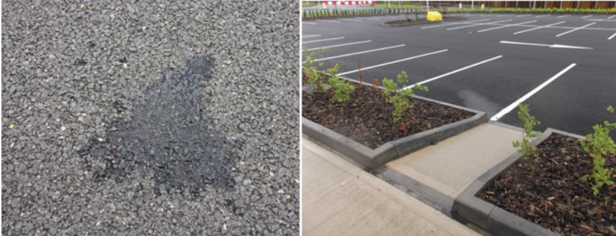
Permeable pavement staff car park (first part of truck access road also drains into this area)
