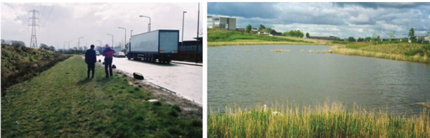
Source control swale, J4M8, connecting with conveyance swale and retention pond
