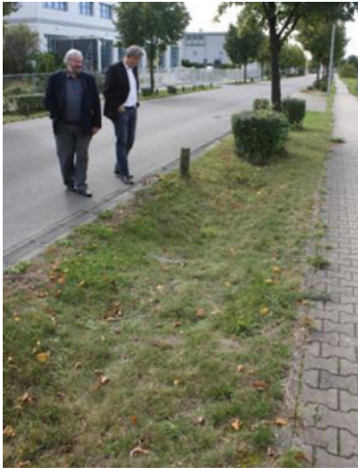
Figure 11.6 Effective drop down kerb line along edge of road, able to feed sheet flow runoff into the under-drained grass swale ( left ) Unfortunately laid line of kerbs on one swale section illustrates risks with good innovations poorly understood by a builder ( right ) Hoppegarten 2014. Photos credit BJ D'Arcy
