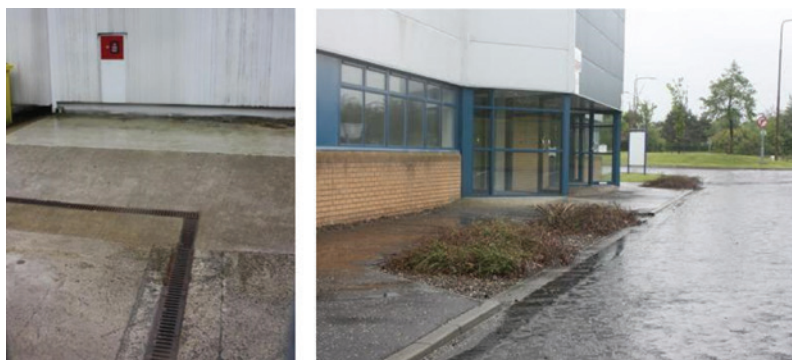
Figure 17.13 Demarcation and collection drain for higher risk outdoor yard area ( left ). Rain garden taking road runoff and providing visible treatment facility with reduced risk of direct contamination of water environment in event of a spill ( right ).
