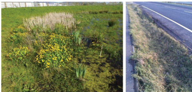
Figure 9.10 Extended detention basin, with source control feeder swale serving service road, Kinross, UK.
