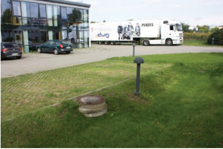
Combination of grassed additional car parking filter strip with grassed detention basin-swale; Hoppegarten industrial estate, near Berlin, Germany
