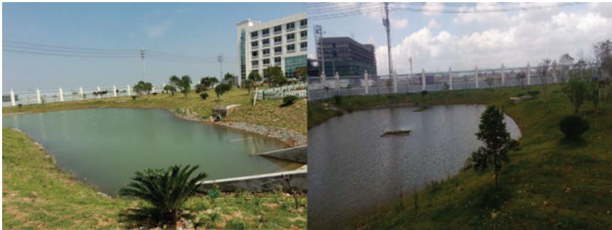
Figure 8.3 Detention ponds in the industrial park. All stormwater from the campus must be discharged to the ponds.
