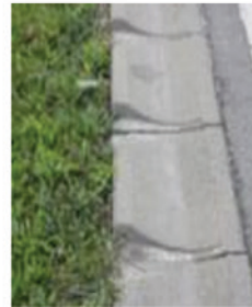
Figure 11.6 Effective drop down kerb line along edge of road, able to feed sheet flow runoff into the under-drained grass swale ( left ) Unfortunately laid line of kerbs on one swale section illustrates risks with good innovations poorly understood by a builder ( right ) Hoppegarten 2014. Photos credit BJ D'Arcy
