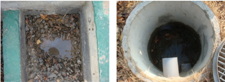
Figure 12.5 Sediment, debris and litter deposition in the sedimentation and facility outlet to drainage access were inspected as part of routine maintenance for the hybrid constructed wetland.
