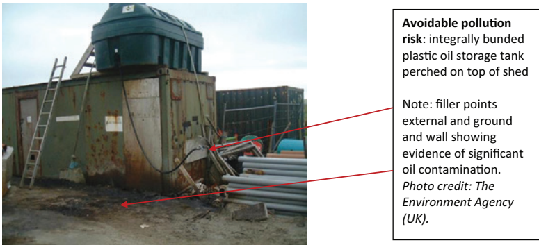
Figure 17.10 An integrally bundled tank that has filler points outside the bund and consequently still presents pollution risks.
