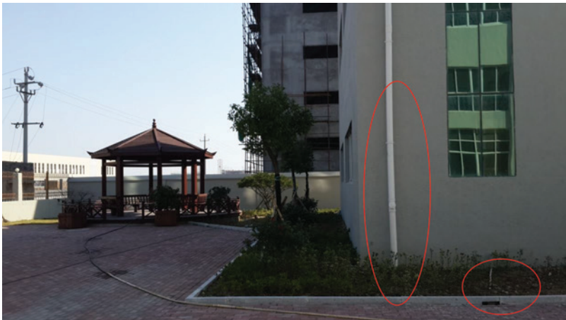
Figure 8.5 Disconnection of roof downspout and rain garden.
