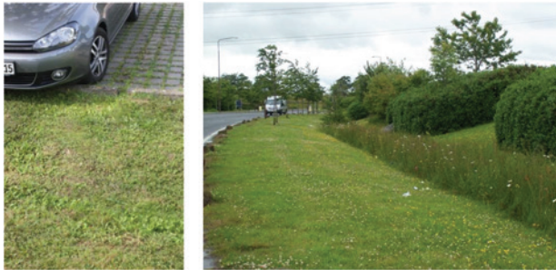
Figure 9.2 Left: Grass filter strip taking car park runoff, Germany. Right: Filter strip draining to conveyance swale, J4M8 distribution centre, Livingston, UK (photo: Chris Pittner).
