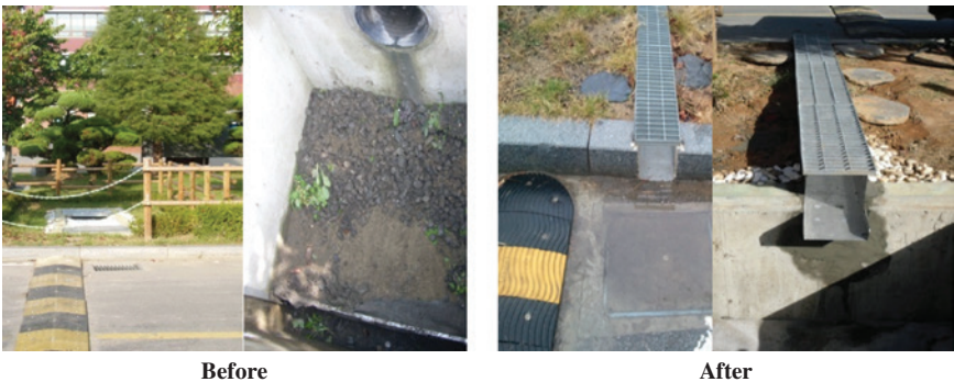
Figure 12.12 The inflow channel of the infiltration trench was renovated as part of the non-routine maintenance.
