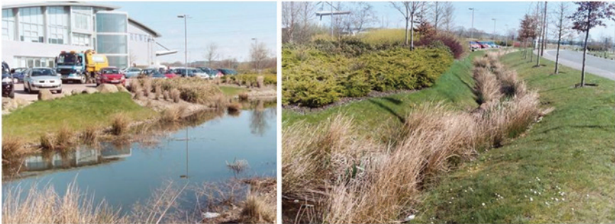
Source and Site controls (filter strip and pool), feeding head of a conveyance swale, J4M8
