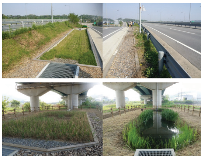
Figure 12.15 On-site photographs of newly-constructed and regularly maintained BMPs in Sejong city, South Korea.
