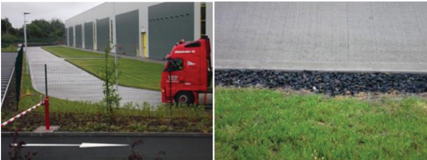
Filter drains at edge of main internal concrete road, taking runoff from truck access route, Dunfermline, Scotland, UK.
