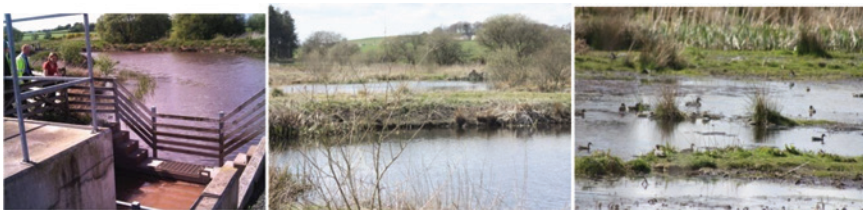
Figure 9.11 Retention pond in modular arrangement (3 ponds and a wetland) receiving runoff from a timber industries business park in Scotland, UK. Note the provision for management of incidents as well as day to day runoff. Swales or filter drains provide the source controls around the site.
