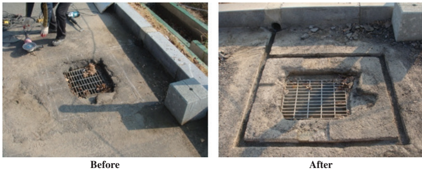
Figure 12.14 A flow diversion channel was constructed to ensure flow diversion to the hybrid constructed wetland as part of the non-routine maintenance.
