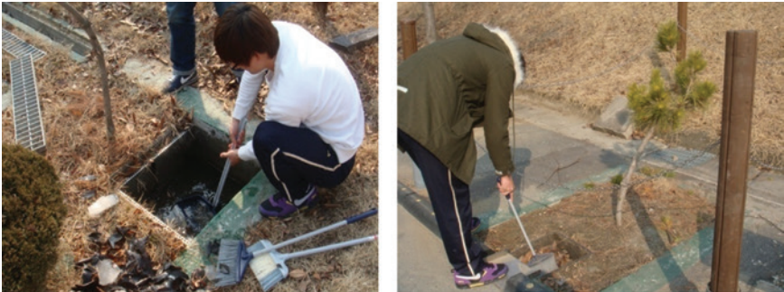
Figure 12.6 After inspection, litters and debris were collected as part of routine maintenance.
