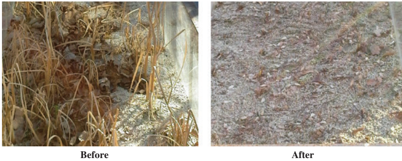
Figure 12.7 Another routine maintenance performed for the hybrid constructed wetland was the management of vegetation and ground cover conducted during the plant dormancy period in winter.
