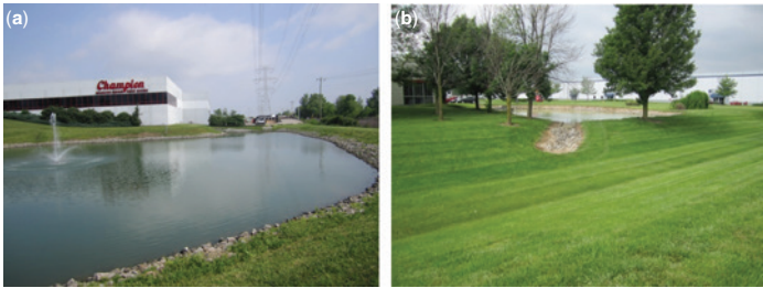
Figure 12.17 Maximizing maintenance costs: conventional design and management of (a) a retention pond ( above left ) and (b) pond and vegetated strips ( above right ) for treating runoff from industrial areas (Cincinnati).
