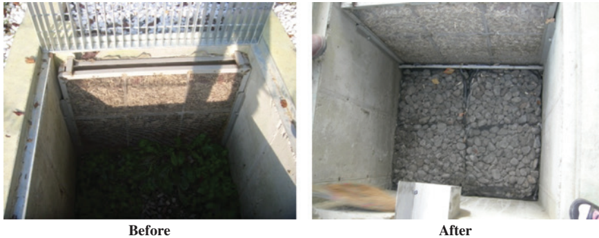
Figure 12.13 Filter media were packed for ease of maintenance in the infiltration trench as part of the non-routine maintenance.
