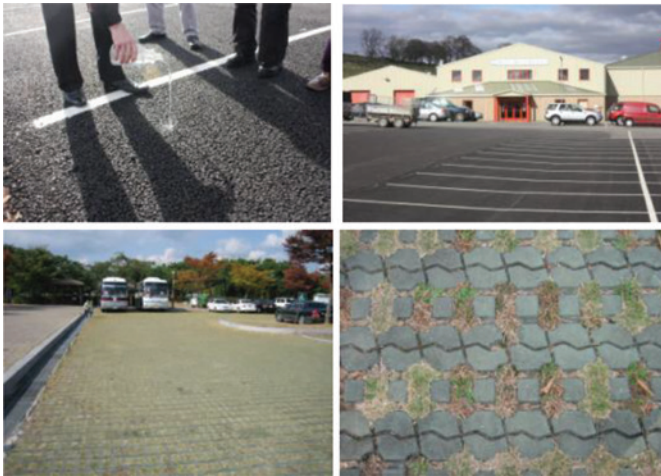
Figure 9.8 Above: Permeable blacktop serving the car park for a meat trading market near Dingwall Scotland, UK. Below: Hybrid concrete/grass permeable surface, with exceedance flow collection drain, serving a coach and car parking area at a water utility installation in South Korea.
