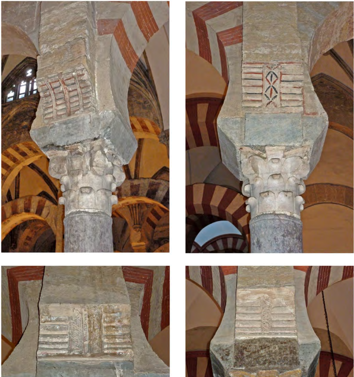
FIGURE 57 Cordoba IV: increasingly decorative roll corbels, some with traces of colour (section 2.1.2.2), and the standard capital used throughout the 'Amirid extension (section 2.1.3.4)
