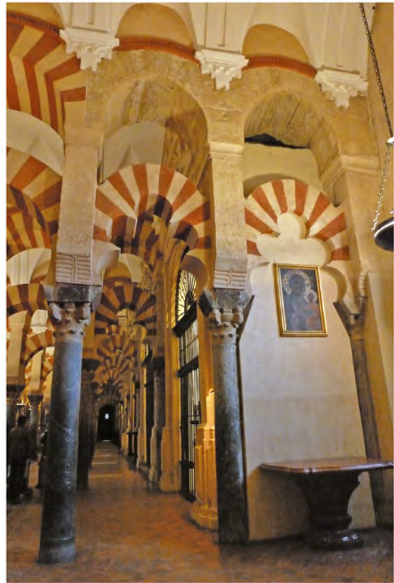
FIGURE 55 Cordoba IV: double bays of lobed arches in the compensating zone along the interior of courtyard façade (section 2.1.1.2)
