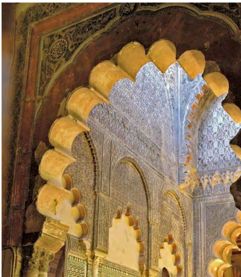
FIGURE 79 Āmirid tribune: 11-lobed arch at southern end. The western double-capital is just visible at the bottom of the photo.
