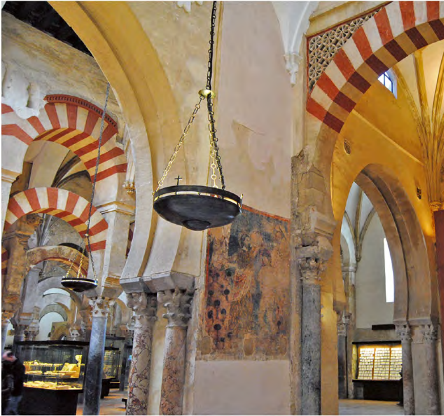
FIGURE 76 Transverse arcade, where it abuts the eastern end of prayer hall, supported by an Āmirid column © CONCEPCIÓN ABAD AND IGNACIO GONZÁLEZ CAVERO
