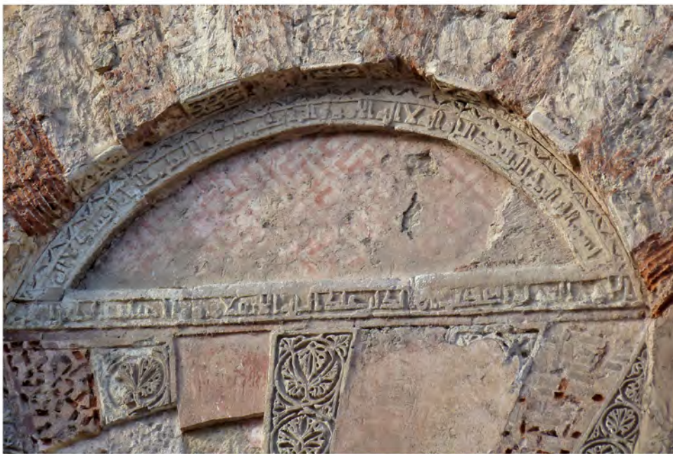
FIGURE 69 Āmirid eastern façade: Gate 2: view and detail of inscription in archivolt © MARIAM ROSSER-OWEN
