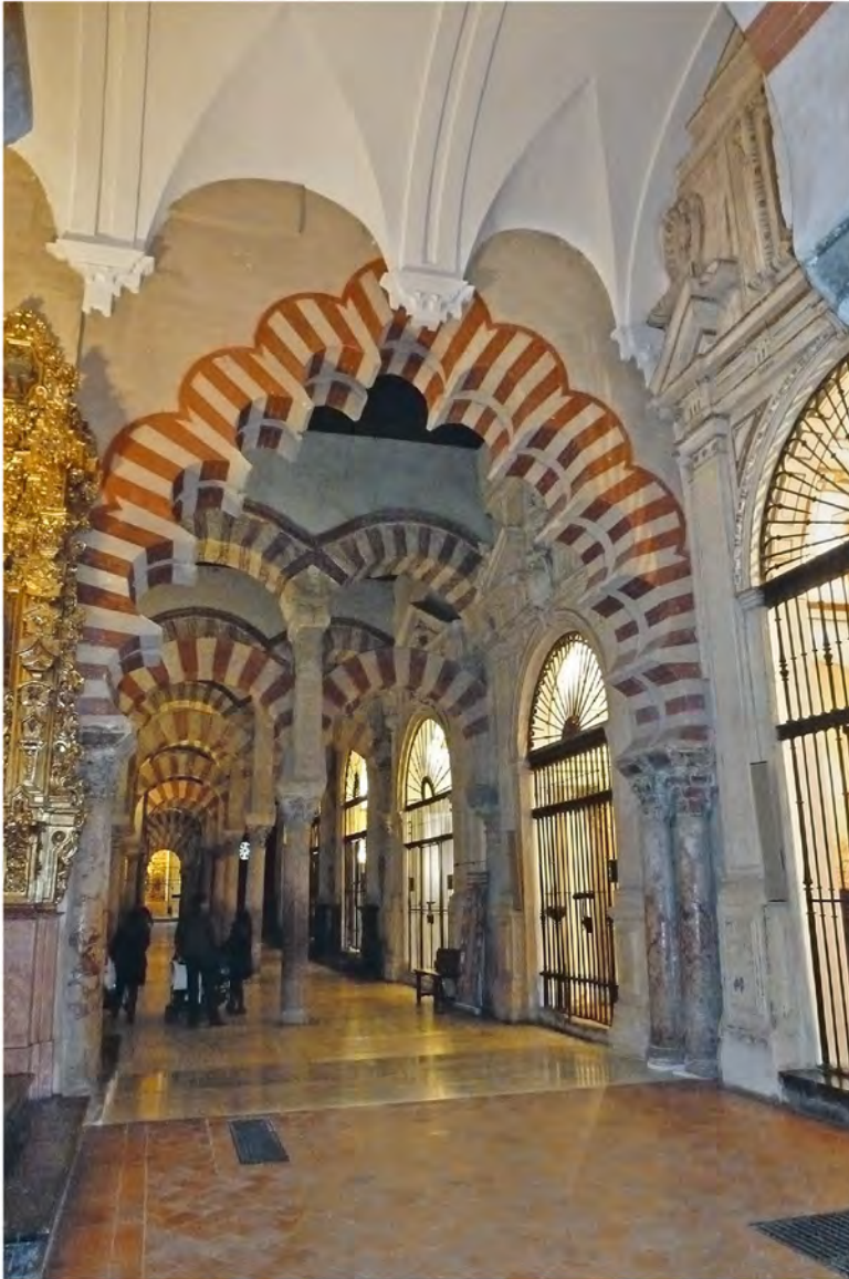
FIGURE 60 11-lobed arch at the junction of Cordoba I and Cordoba IV, terminating the longitudinal arcade (section 2.1.3.2)
