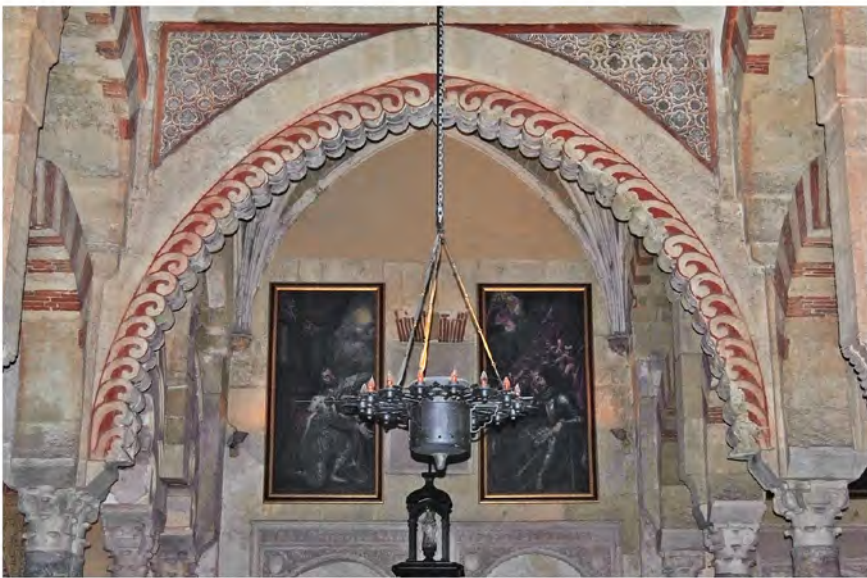
FIGURE 77 Transverse arcade along the qibla wall: arch to the west of maqṣūra naves, with rolls in intradoses © CONCEPCIÓN ABAD AND IGNACIO GONZÁLEZ CAVERO
