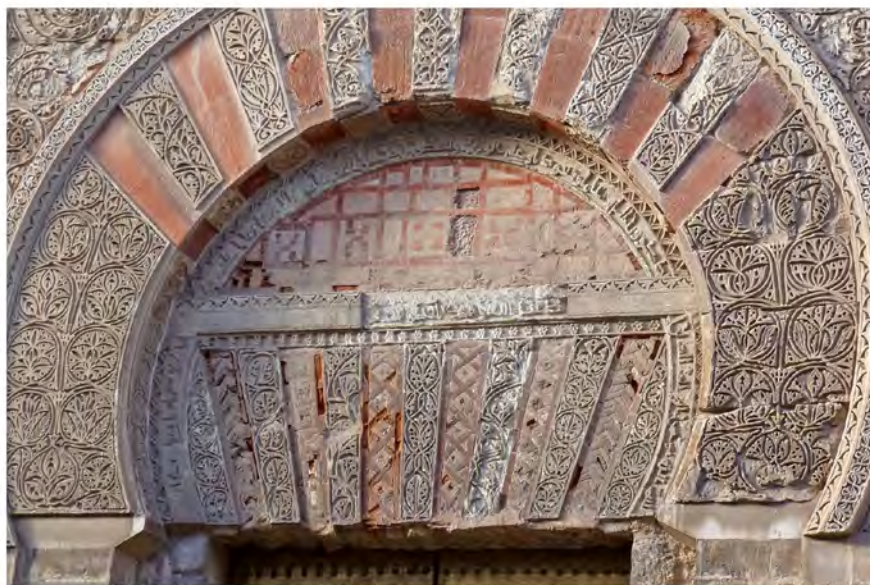
FIGURE 74 Āmirid eastern façade: Gate 7: view and detail of inscription in archivolt © MARIAM ROSSER-OWEN
