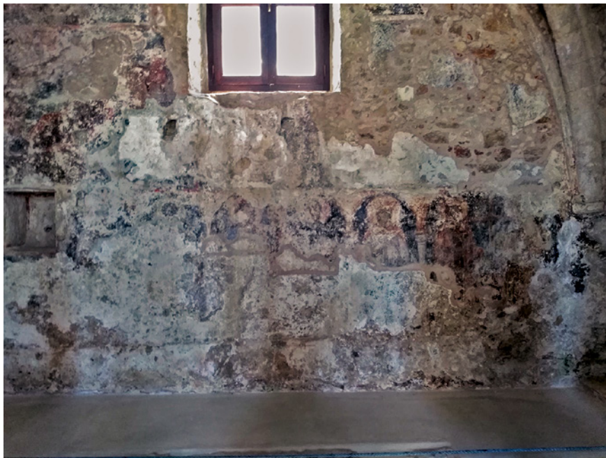
FIGURE 79 Traces of wall paintings in the south chapel of the conventual church of St Peter the Martyr, Heraklion
