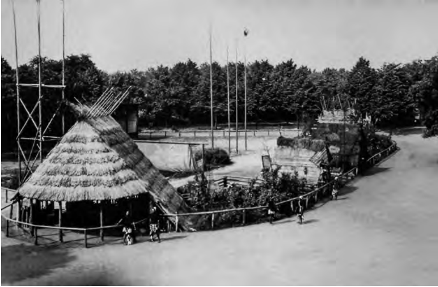
Figure 2.4. A rare photograph of an ethnic show village under construction. The erection of houses with thatched roofs and of a temple structure in the background around wooden or metal poles are clearly discernible. Indian-Ceylonese performers are visible in the foreground. Postcard. Private collection of Hilke Thode-Arora.
