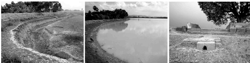
Figure 6.2 Budhauri Ahar in February (left) and August (middle), 2016 and its Outlet (right)
