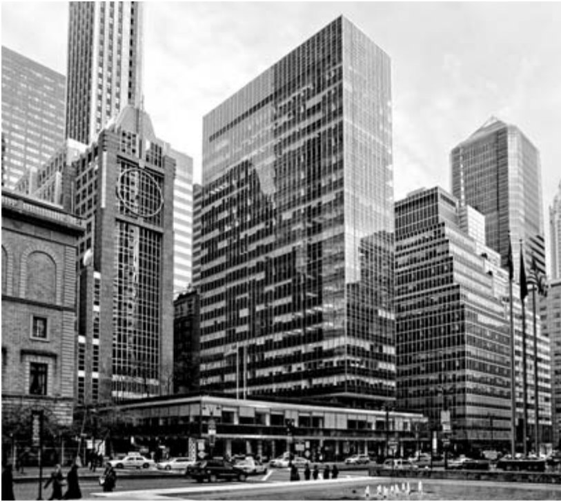
FIGURE 2.2. The Lever House at 390 Park Avenue, New York, a well-known example of International Style architecture. Architect: Gordon Bunshaft for Skidmore, Owings, and Merrill, 1952. Photograph courtesy of Nathaniel Robert Walker.
