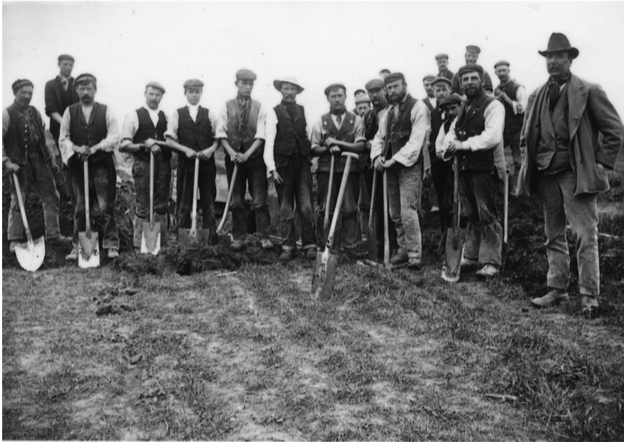
A gang of navvies near Haddenham, Buckinghamshire take time off from their work on the Great Western & Great Central
