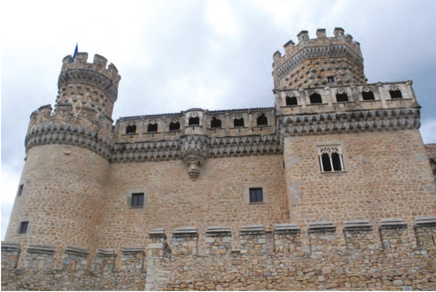
FIGURE 14.10 Castle Palace of Manzanares el Real. Andamios at the top of the wall, last quarter of the 15th century PHOTO: AUTHOR
