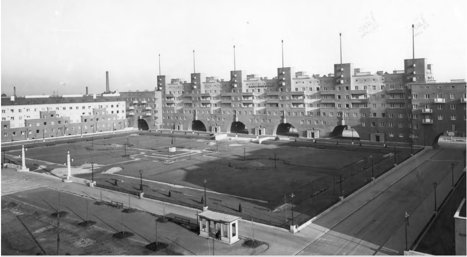
Fig. 127: The forecourt and central tract of the Karl Marx Hof in Vienna around 1930. Source: Municipal and Provincial Archives of Vienna, 3.3.2.FC1.2961M.
