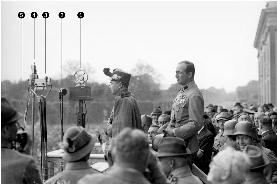
Fig. 107: Engelbert Dollfuß (at the microphones) and Ernst Rüdiger Starhemberg (behind him) on the garden terrace of Schönbrunn Palace in Vienna at the “Turks Deliverance Celebration” on May 14, 1933 (numbers added): ❶ carbon microphone (model unknown); ❷ dynamic microphone (probably a Western Electric 618A); ❸ carbon microphone (Reisz); ❹ carbon microphone (Reisz) and above it a dynamic microphone (model unknown); ❺ possibly a microphone by the Selenophon Licht- und Tonbild GmbH. Source: Austrian National Library, 106.661 B
