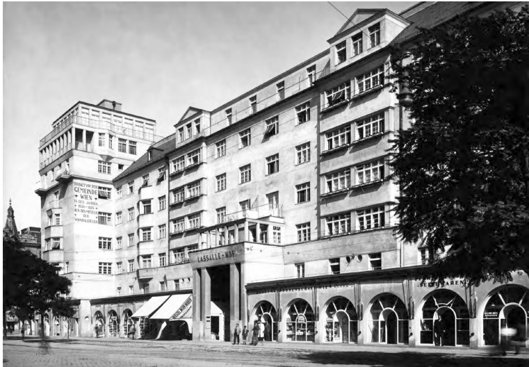
Fig. 105: The Lassalle Hof in Vienna, photographed from the Lassallestrasse in 1926. Source: Municipal and Provincial Archives of Vienna, 3.3.2.FC1.407M.
