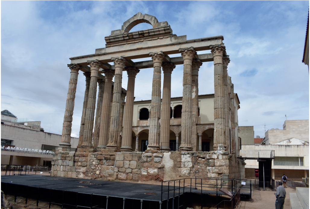
Figure 13.2. Concrete structures around the Temple for the Imperial Cult, the new 'forum' of Mérida (author).
