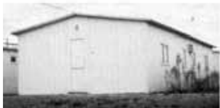
Figure 2 Temporary shelters in Izmit (Baradan, 2002, p. 93)
