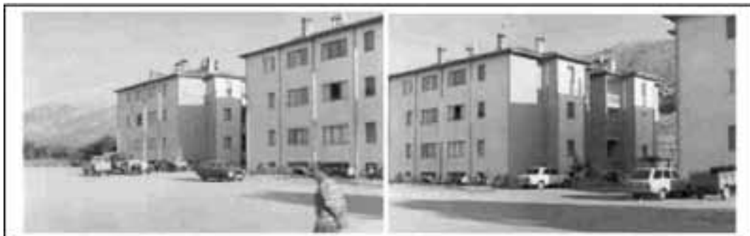
Figure 2. Exterior views of the Ikitelli post-disaster housing settlement.
