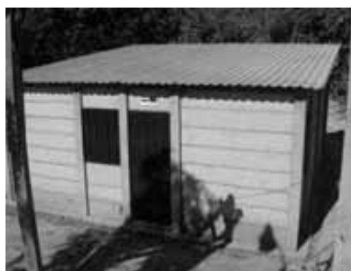
Figure 2. RC Prefabricated house
