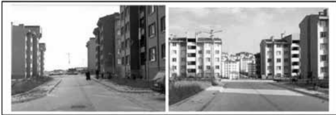
Figure 1. Exterior views of the Ikitelli post-disaster housing settlement.
