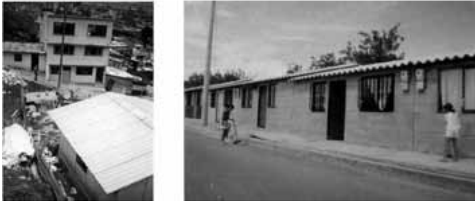
Figure 2. Left : Informal settlement in Bogotá showing 4 different stages in the housing evolution process: from a shack made of scrap wood to a three storey unit made of concrete and masonry. Right : 1-storey units in El Cantarito. Despite that higher densities were obtained and infrastructure was provided, few months after the project was finished, users had already modified the rigorously standardized facades to personalize them with colours and finishes.
