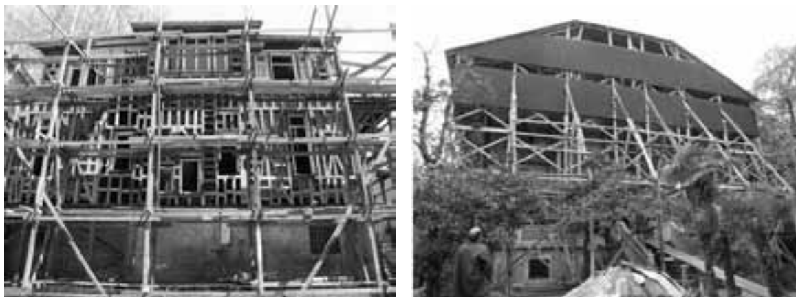
Figure 10. Temporary consolidation of the timber frame structures (Can Binan's archives).
