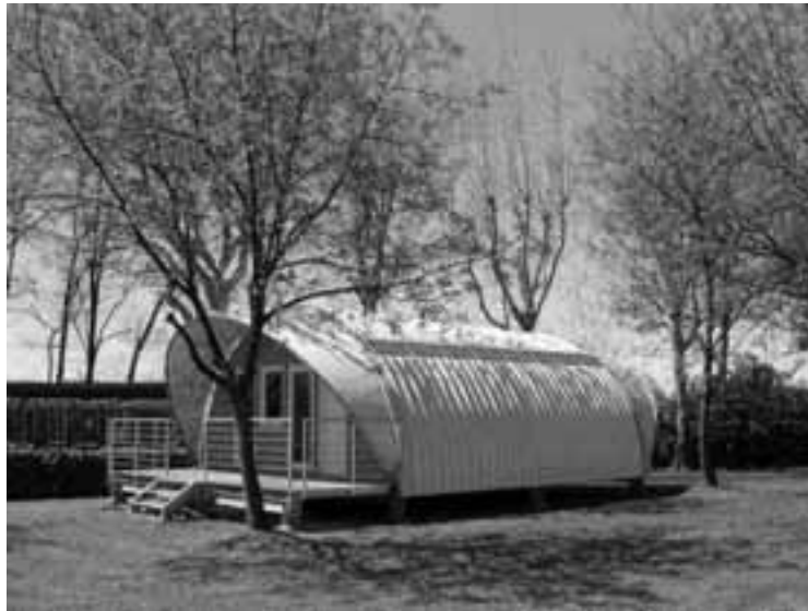
Figure 1. Prototype of L'Armadillo in Carate Brianza (MI) integrating photovoltaic cells on the top.
