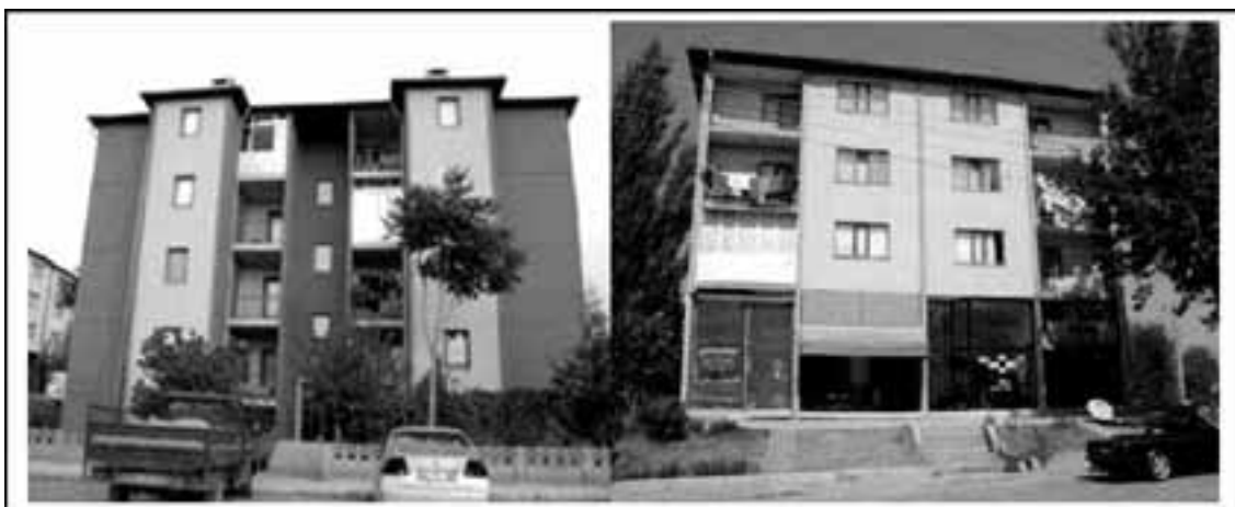
Figure 1. Two types of post-disaster houses in center of Dinar .
