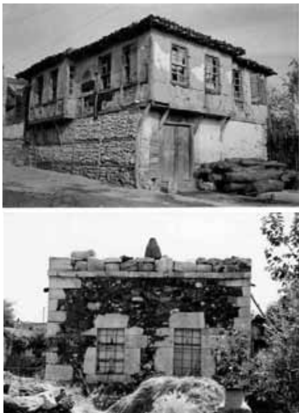
Figure 5. The timber frame construction with masonry infill and masonry construction examples of traditional houses.
