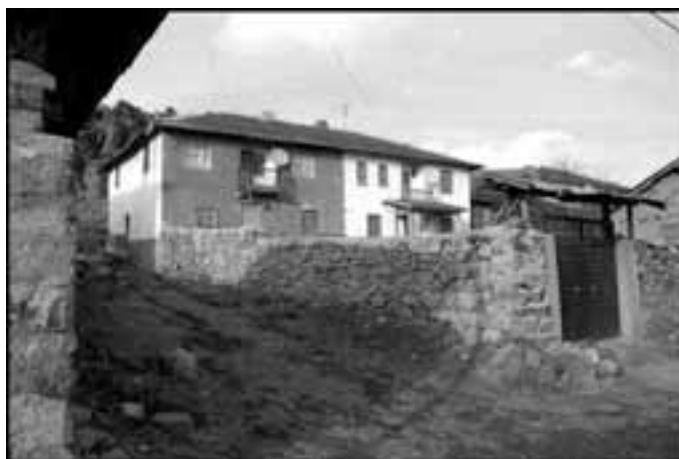
Figure 2. A house in old Yuva Village.
