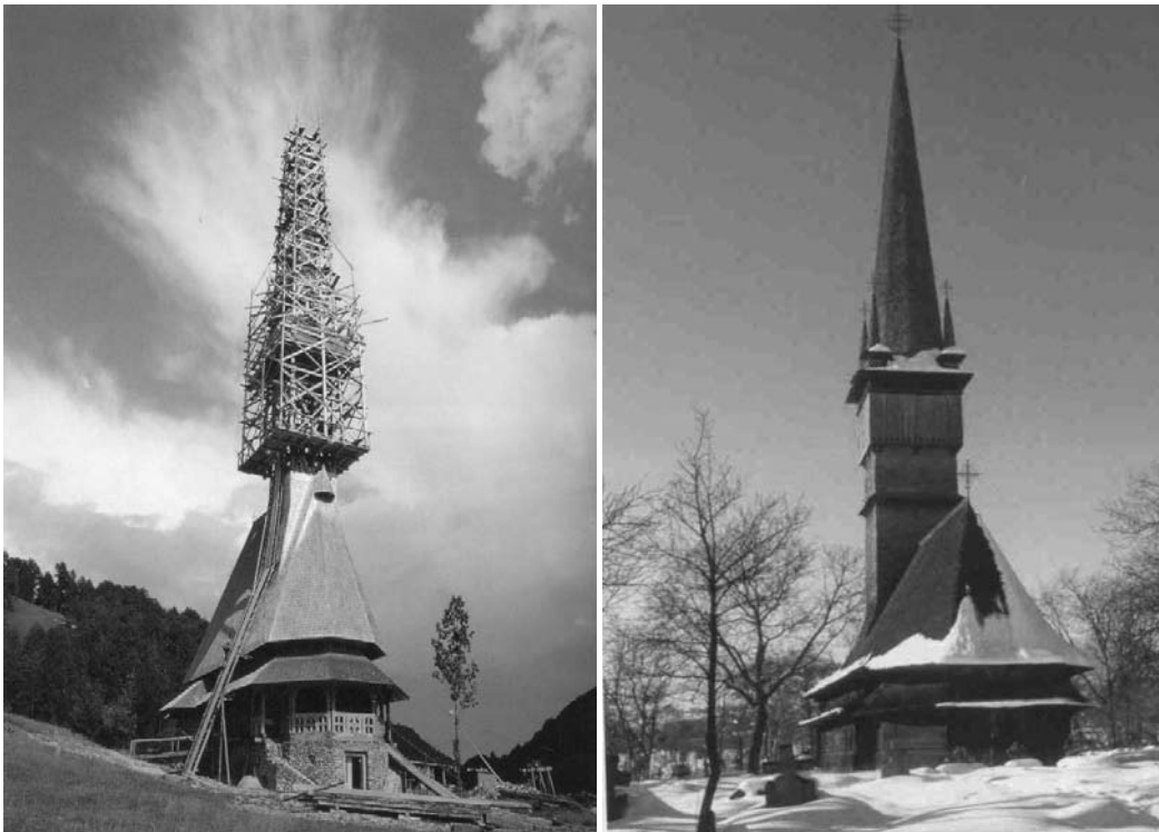
Fig. 3 Maramureș wooden church during and after repair
