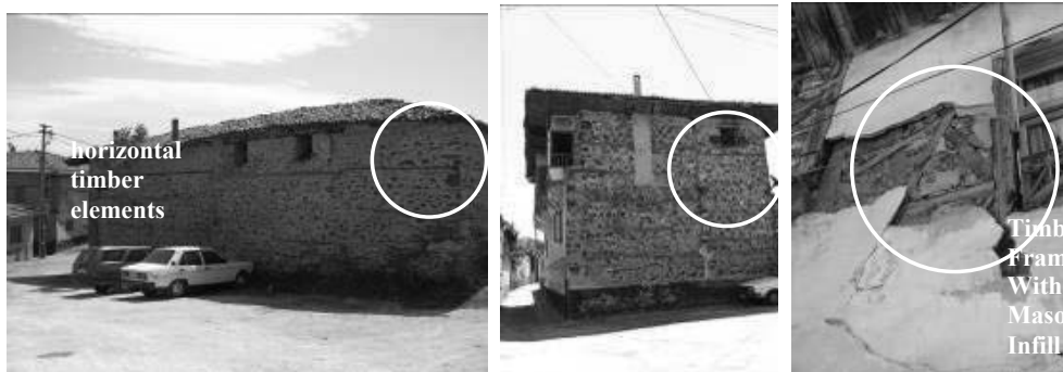
Fig. 2: Construction System of Kula Traditional Houses
