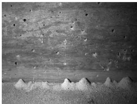
Fig. 12. Frass at construction
