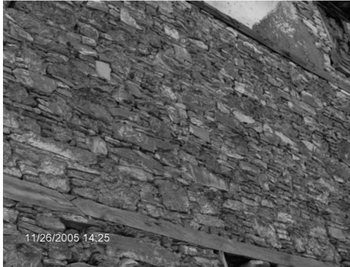
Fig. 1: Horizontal Timber Lintels
