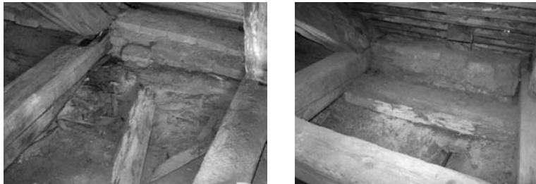
Fig. 8. Attack of the insects ( Hylotrupes bajulus L.)
