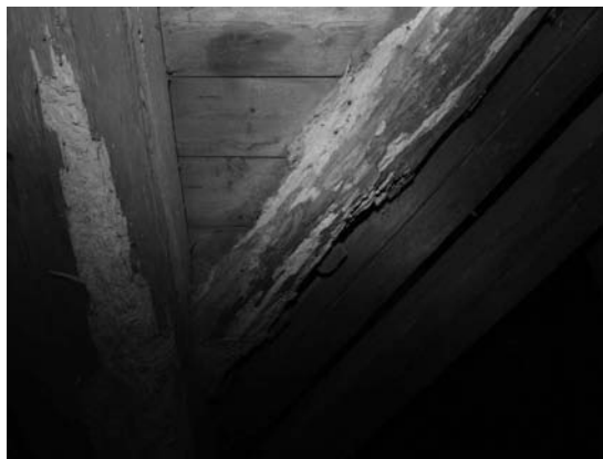
Photo 2 Beetle attack in the old church in Ruhnu
