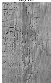
Fig. 7 – Damages by woodboring anobiid beetles.
