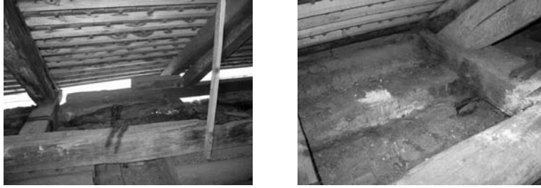
Fig. 6. Restoration of the roof cover without replacing damaged supporting elements.
