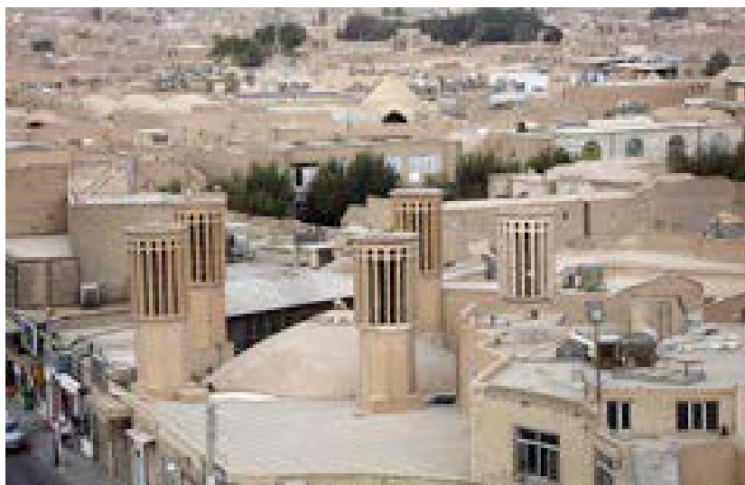
2. Iran, edificio urbano con cupola e torri del vento 2. Iran, urban building with cupola and wind towers
