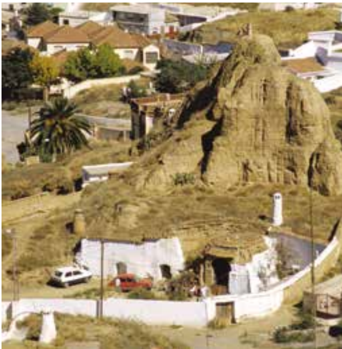
Fig. 1 Cave dwelling excavated on the slope of a promontory in Guadix, Spain (photo: F. Vegas and C. Mileto).
