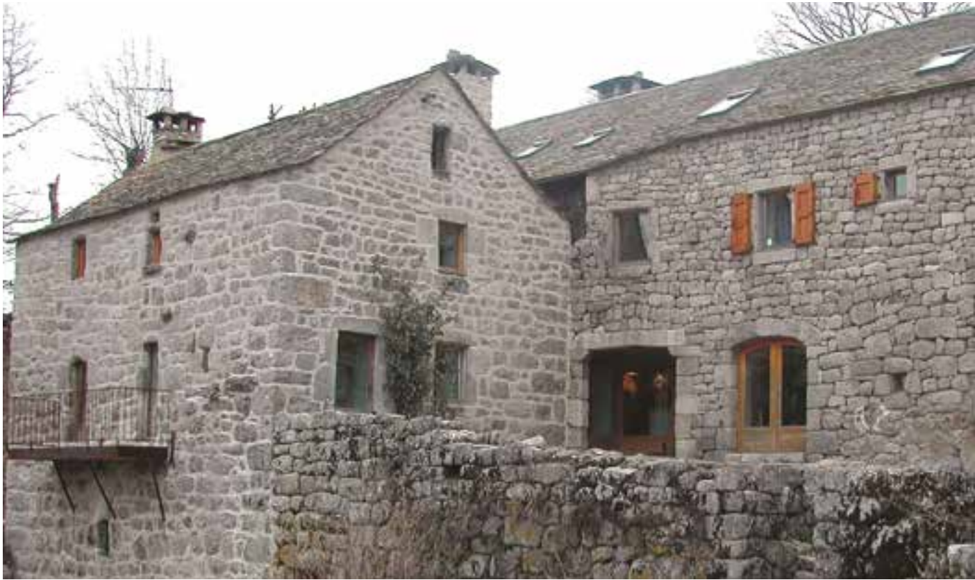
Fig. 1 Roof in lauzes (stone-slates) at Le-Pont-de-Montvert, Cévennes, France (photo: H. Guillaud).
