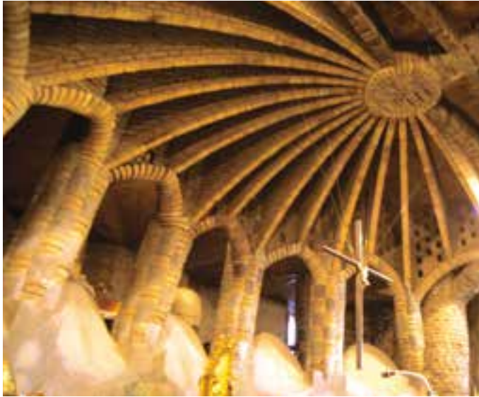
Fig. 7 Gaudí's buildings show that personal creativity and new architectural shapes are not at odds with using traditional techniques. Cripta Colonia Güell vault, Barcelona, Spain (photo: F. Vegas, C. Mileto).
