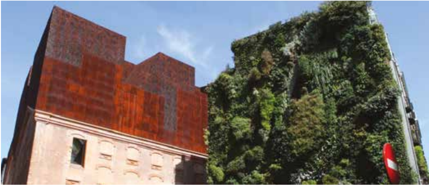
Fig. 3 Caixa Forum building in Madrid by Herzog and de Meuron, with its vertical garden designed by the French botanist Patrick Blanc (2008). Madrid, Spain (photo: L. Dipasquale).
