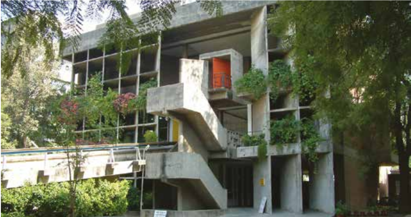
Fig. 23 Millowner's Association building by Le Corbusier, with its characteristics brise-soleils to prevent the hard sun from entering inside. Ahmedabad, India (photo: F. Vegas, C. Mileto).
