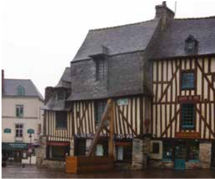
Fig. 3 Timber framework house in Normandy, France (photo: L. G.F. Cannas).
