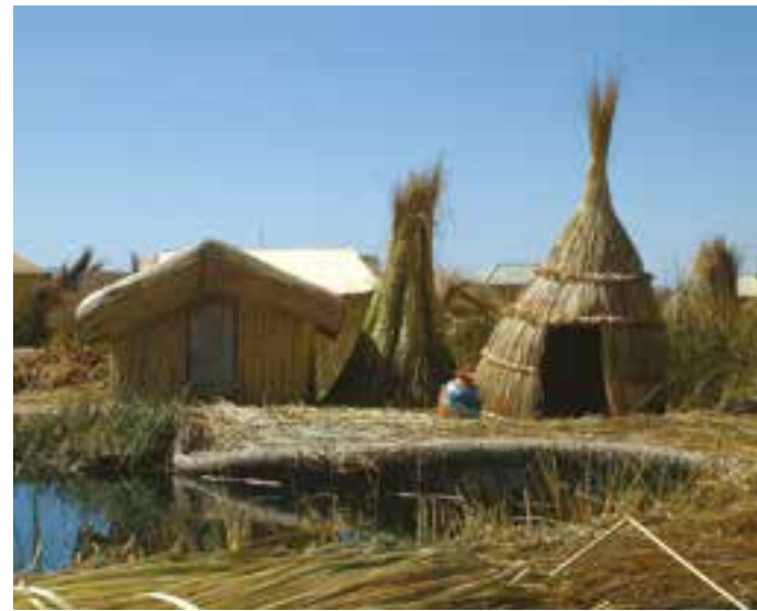
Fig. 4 Floating totora reed dwelling of the Uros people on Lake Titicaca (photo: F. Vegas, C. Mileto)
