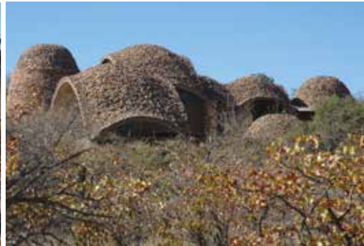
Fig. 12 Mapungubwe Interpretation Centre by Peter Rich Architects (2009). Limpopo, South Africa. (photo: P. Rich)
