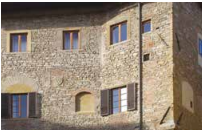
Fig. 4 Anchor plates in a stone building in Florence, Italy (photo: L. Dipasquale).
