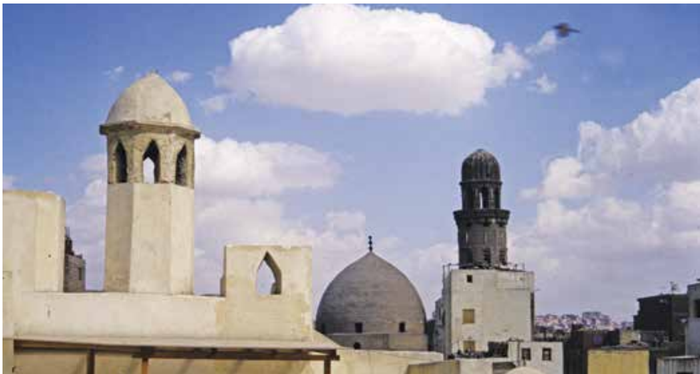
Fig. 22 Vents on top of stairways and domes that generate the circulation and renewal of fresh air in the dwellings. Cairo, Egypt (photo: F. Vegas, C. Mileto).
