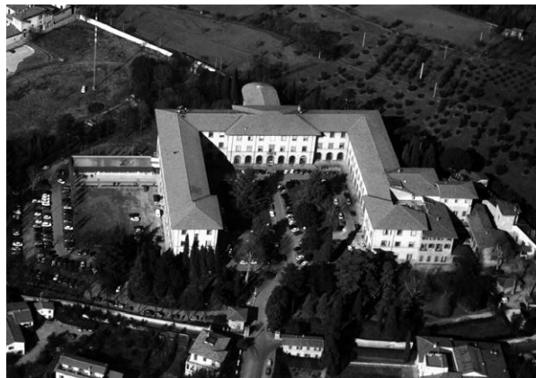
Fig. 1 – Aerial view of S. Marta complex, the historical building of the School of Engineering of Florence.
