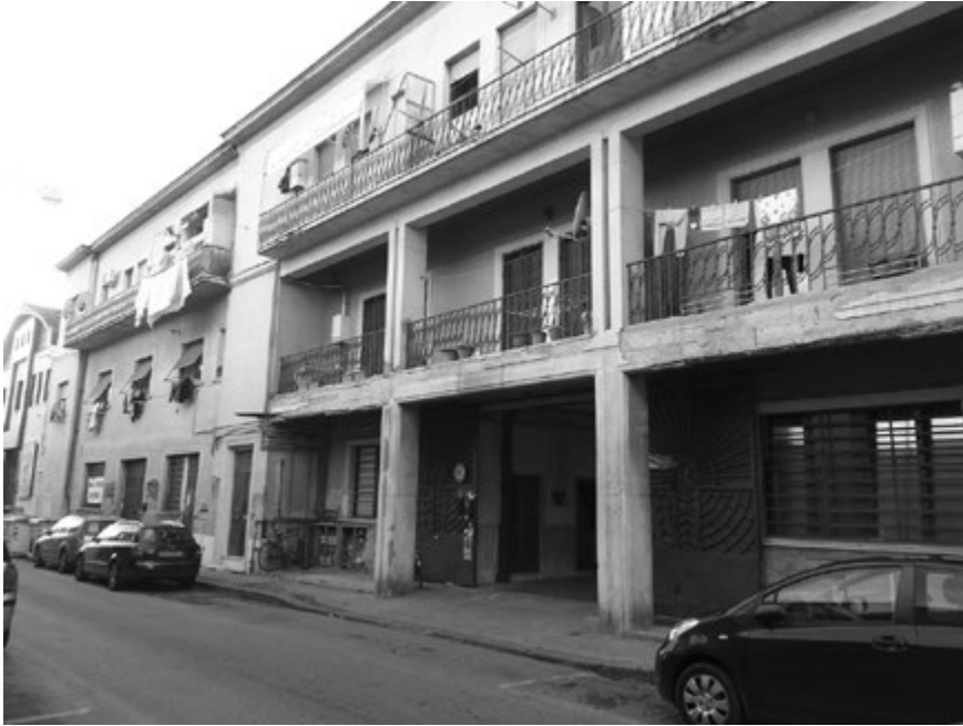
Figure 3. A building shared by multiple stitching workshops in Macrolotto 0 (taken by author on 11/9/2013).
