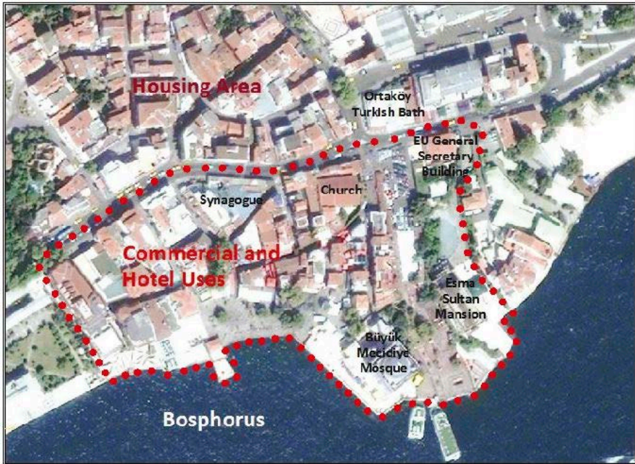
Figure 2 – Aerial photograph of Ortaköy waterfront.
