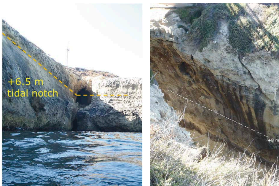
Figure 4 – Past marine markers along the coastal cliff: on the left, the ancient tidal notch at +6.5 m a.s.l. and the entrances of Fungo Cave; on the right, the +8 m a.s.l. lithophaga boreholes band.
