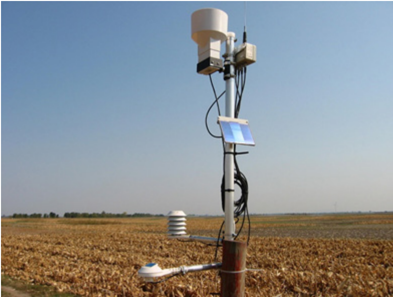
Figure 13.4: Example of a commercial automatic and solar-energy driven agrometeorological weather station for measurement of standard meteorological elements and online data transfer; (Source: BOKU-Met).
