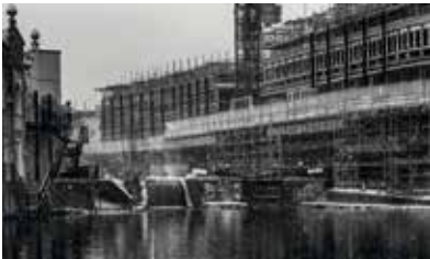
Figure 5. Lock and Building in Progress
