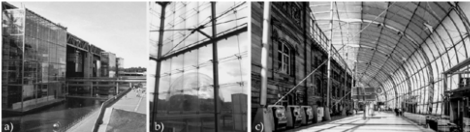
Figure 1.2 - a) & b) Cité des Sciences et de l'Industrie greenhouses and reception, Parc de la Villette, Paris, RFR 1986 c) new TGV railway station in Strasburg, RFR-SNCF 2007
