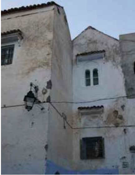
→ Andalusian timber roof External view
