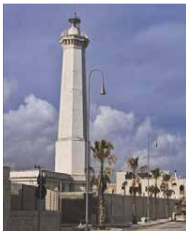
Figure 1 - The Lighthouse of Torre Canne before the restoration works. (Source: Ivona, 2010).
