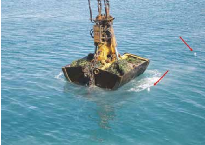
Figure 7 - The red arrows highlight the presence of the buoys which signalled the exact area where to deposit the clod.
