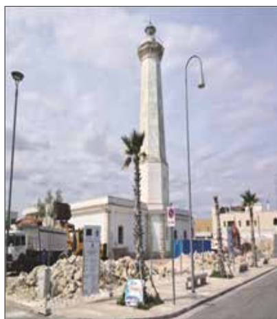
Figure 2 - The Lighthouse of Torre Canne after the restoration works. (Source: Ivona, 2016).
