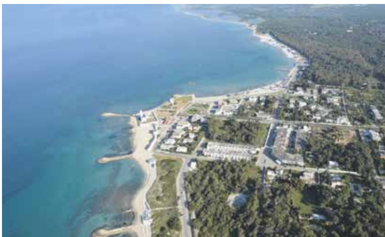
Figure 9 - San Cataldo (Lecce, Italy): north aerial view (LabTAF, 2013).
