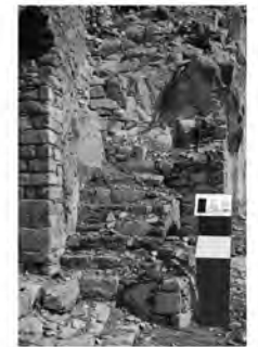
VIEW OVER THE STAIRCASE NEAR THE FURNACE
