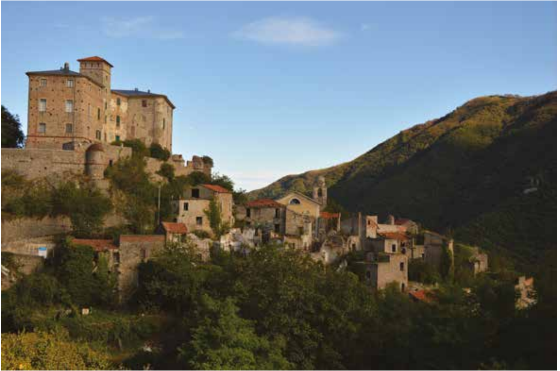
Fig. 1-2 The abandoned village of Balestrino - general view and the church square - Photo Martina Canziani.
