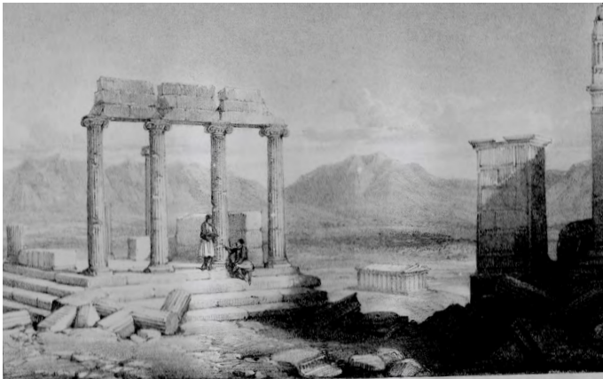
Figure 21.4. The temple to Athena Nike in the course of being rebuilt, February 1836. Lithograph. 22
