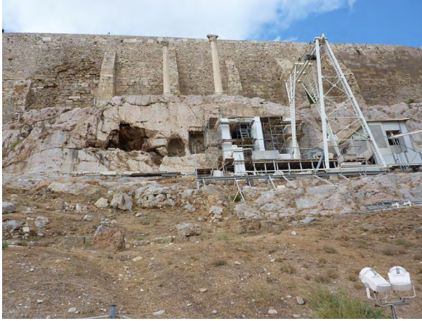
Figure 17.1. The Monument of Thrassylos under restoration 2013. 24
