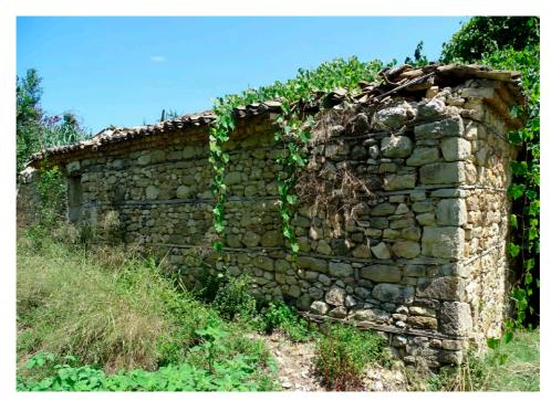
Figure III-4.2 Remains of a traditional dwelling in the hill quarter with horizontal reinforcing timber elements.
