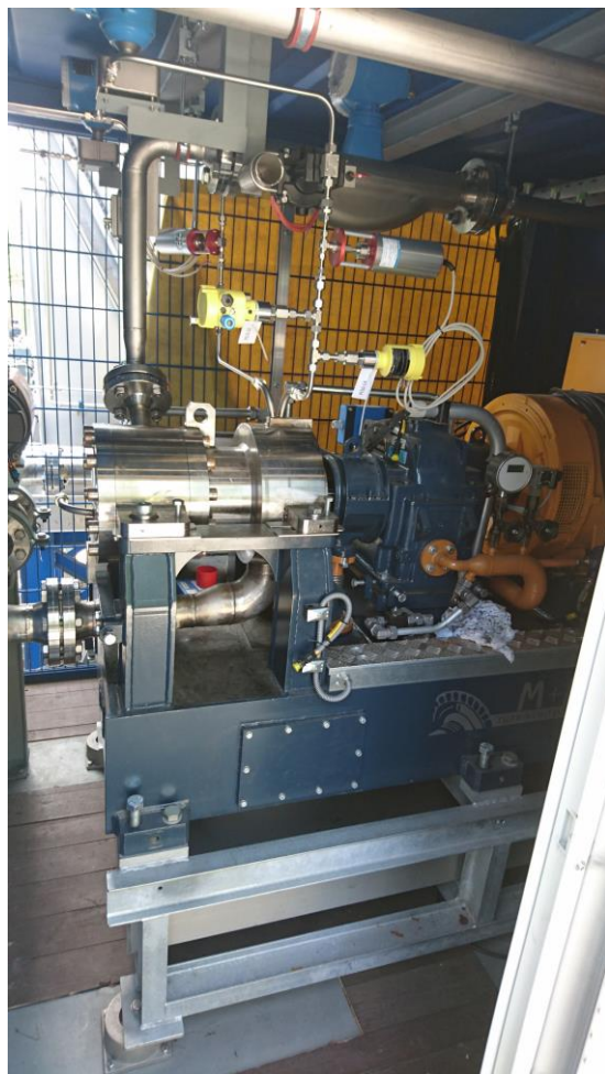
Fig. 5: Turbine with gearbox and generator
