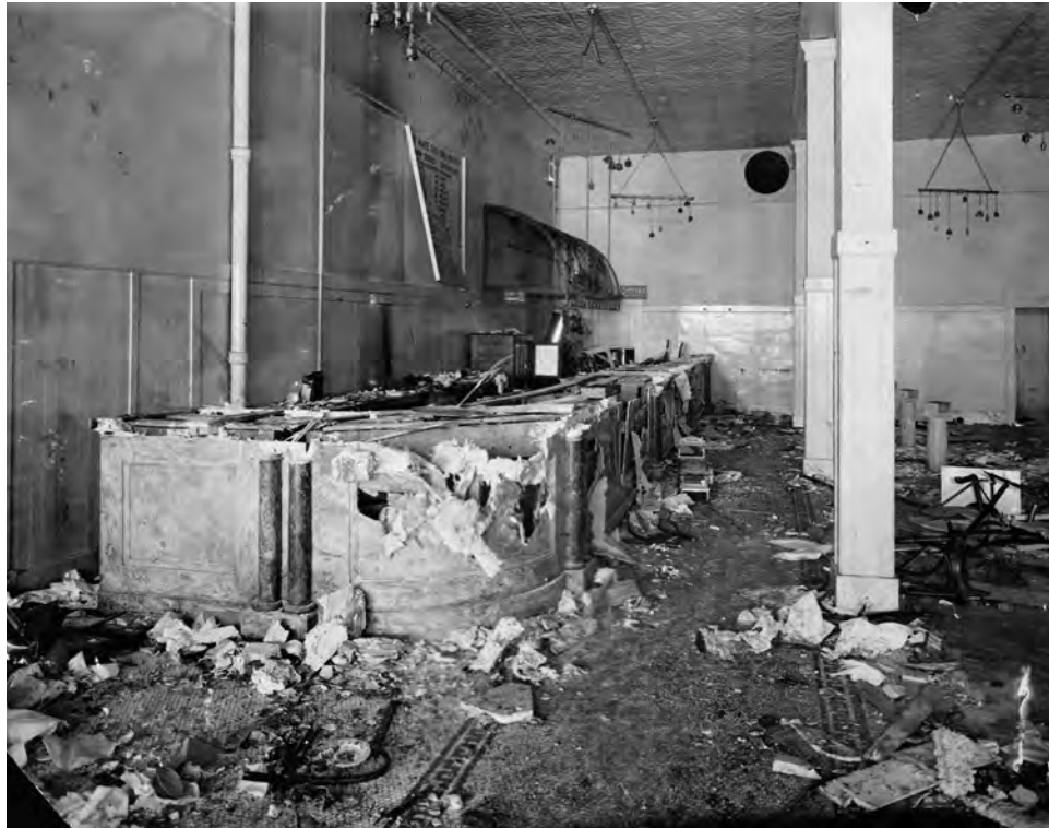
Interior of the Riverside Hotel showing damage, 10 February 1916. Glenbow Archives, NA-3965-11.
