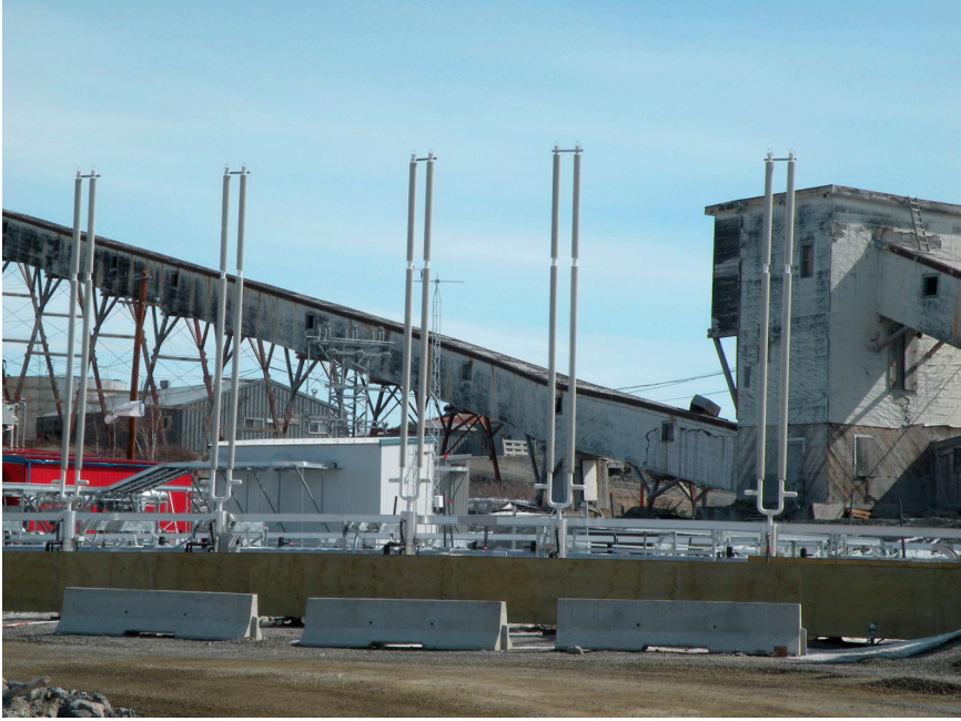
FIG. 11.3: Thermosyphon test plot, Giant Mine Remediation Project. Photo by John Sandlos.
