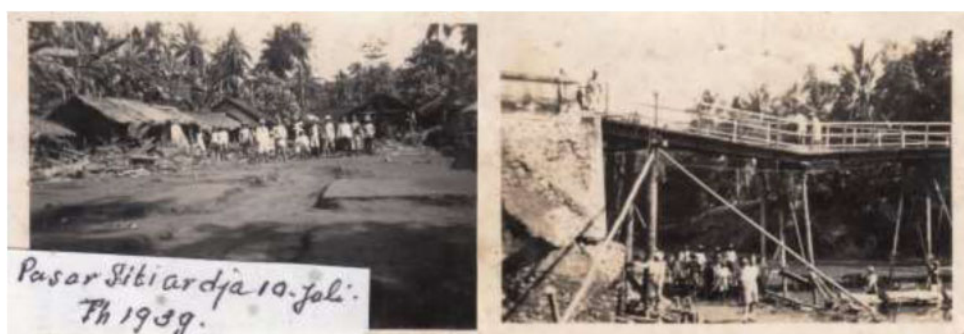
Figure 3. Sitarjo Bridge was destroyed by flash floods, 1939. (Source: Archive Collection of Yusak Khrisyanto).
