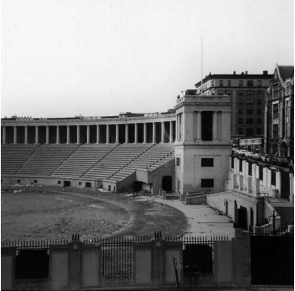
The Lewisohn Stadium in September 1973, a few days before its demolition
