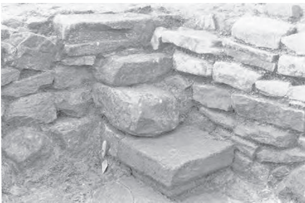
Figure 8.3 The steps down to the courtyard water tank with the reused eaves drip corner stone at the top and an upturned column or pier base at the bottom.
