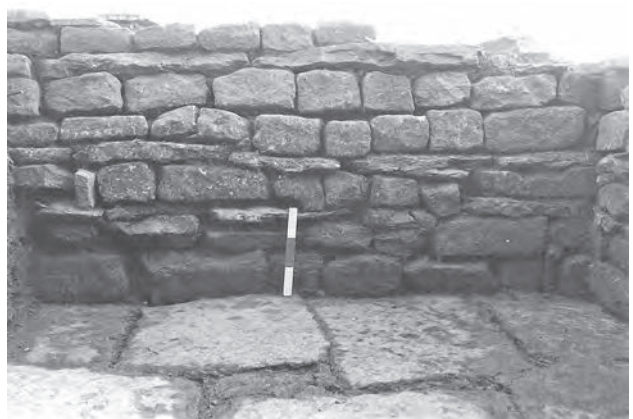
Figure 9.08: South wall of the courtyard cistern (N11:11).
