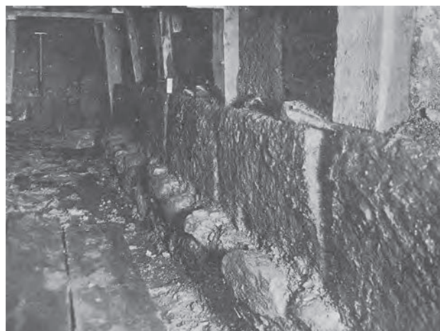
Figure 17.04: Hadrian's Wall curtain at the point where it joins the west gate, looking east. Seen in the tunnel beneath Buddle Street excavated by F. G. Simpson in 1929 (Simpson et al. 1930, fig. 7).
