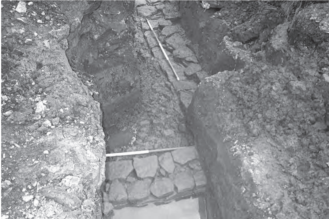
Figure 2 View from the east of the walls of the building uncovered beside Carville Road, north of Hadrian's Wall, in 2006
