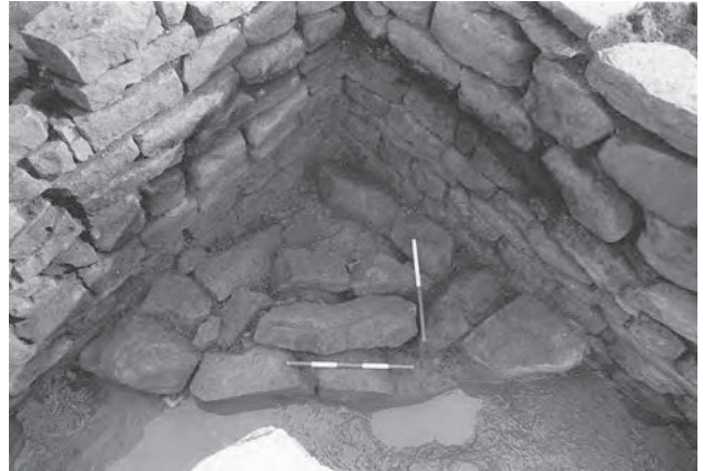
Figure 7.09: Base of the corner buttress, from the north-west.
