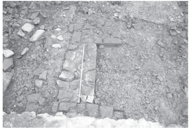
Figure 10.22: The north east corner of the forehall wing gutter K08:19/L08:35 packed with clay (K08:08/L08:21) in front (left) of Piers 1 and 2 and infill wall K08:06/L08:16, looking east (A).
