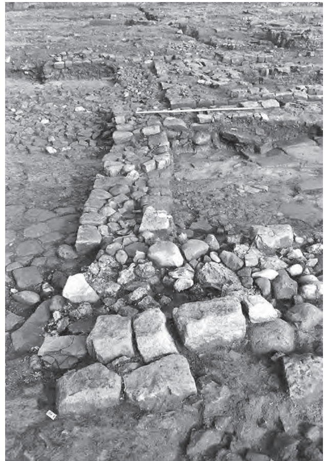
Figure 16.35: Spine wall M14:09 (foreground) north-south wall M14:02, M14:03 separating AL2 (w and e) and rubble foundation of AL2 (e) south wall M14:03 looking east.
