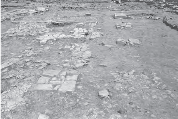
Figure 8 The east portico with Phase 1 (to right) and Phase 2 (centre) column/pillar bases apparent, looking north
