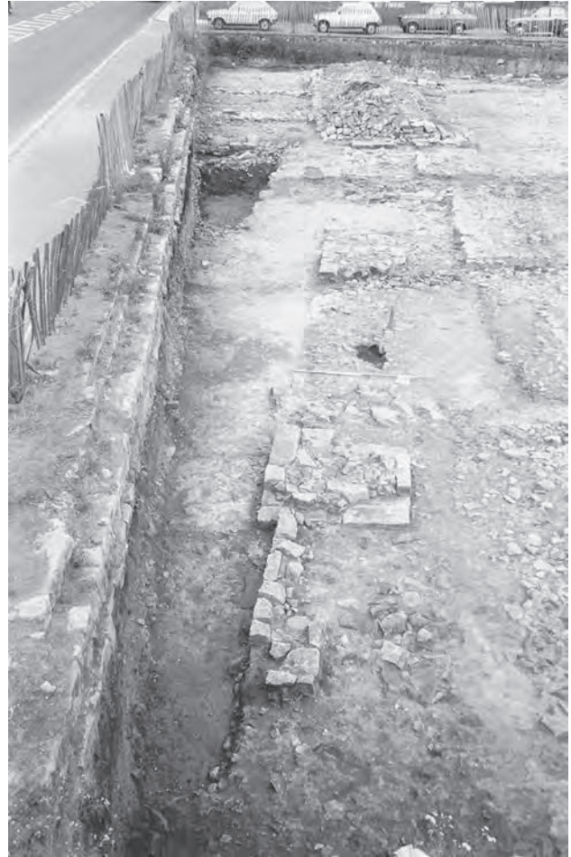
Figure 10.13: Piers 11 and 9 and infill wall G07:05 with the site of pier 1 in the foreground looking east in 2003.
