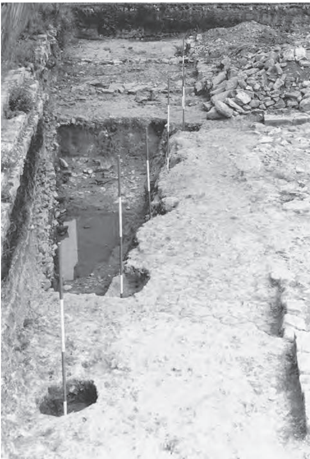
Figure 10.16 Postholes of the forehall portico cut by rectangular pit C2 (shown completely emptied) from the west (Fig 10.16).
